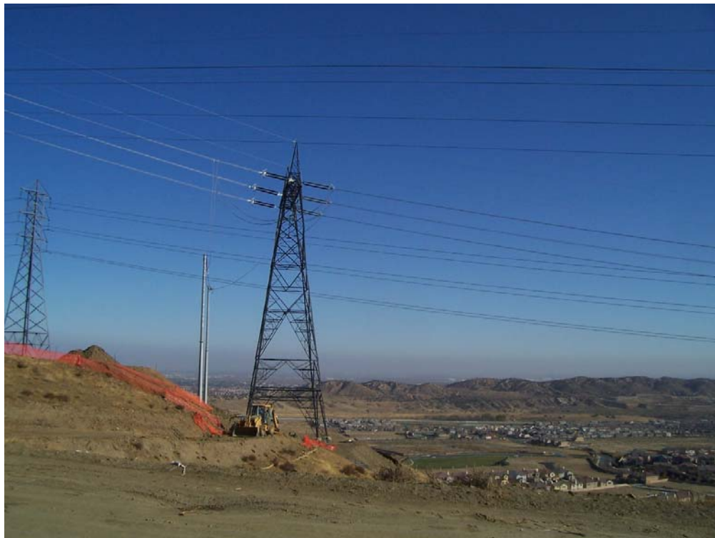
Figure 2: Fiber optic cable installation Towers 79-76, Segment 2.
