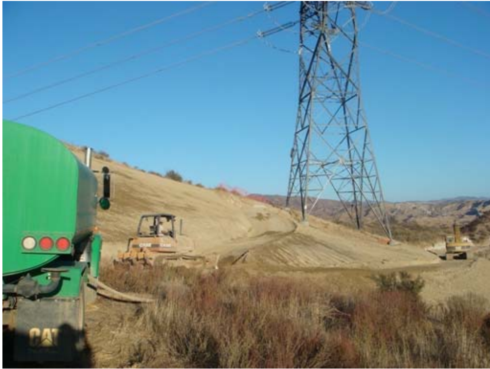
Figure 1: Final road recontouring at Tower 26 A-C, Segment 1.
