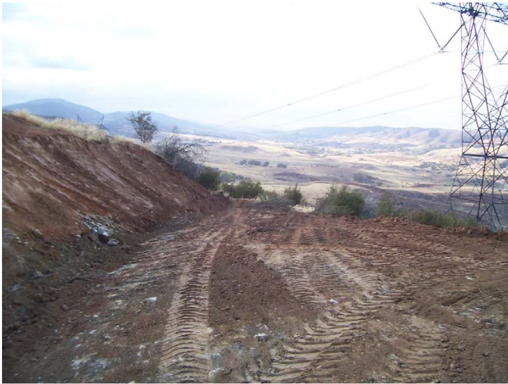
Figure 3: Segment 2 road recontouring at Tower 44.
