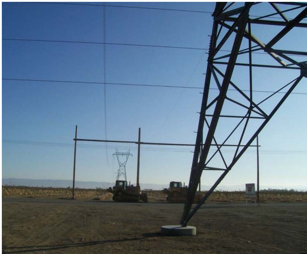
Figure 4: Wire stringing activities between Towers 49-59 Segment 3A.
