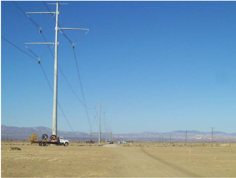
Figure 3: Segment 3 wire stringing activity between Towers 70-71.
