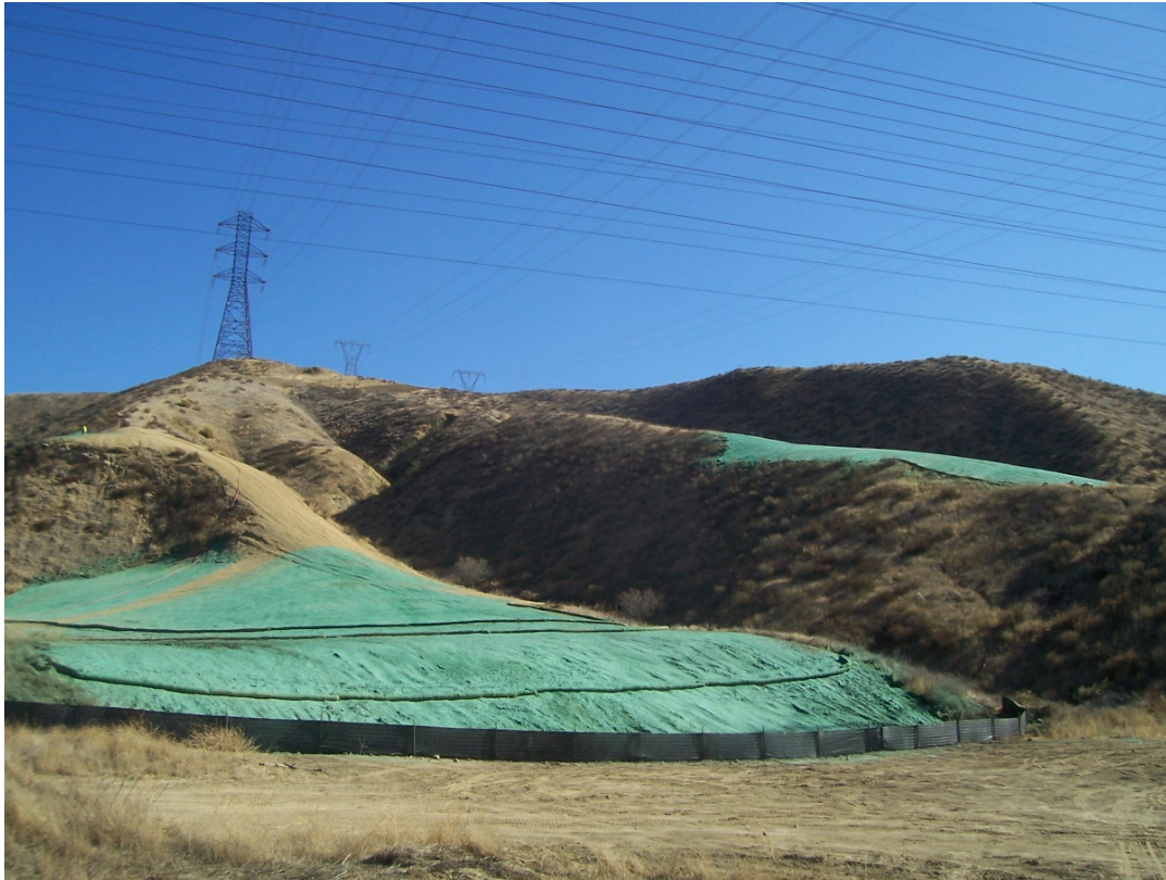
Figure 1: Hydroseeding disturbance areas in Haskell Canyon near Tower 23, Segment 1.
