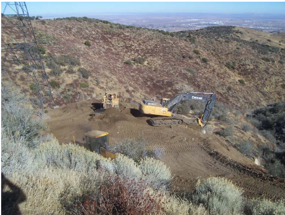
Figure 2: Recontouring project disturbance areas at Tower 59, Segment 2.
