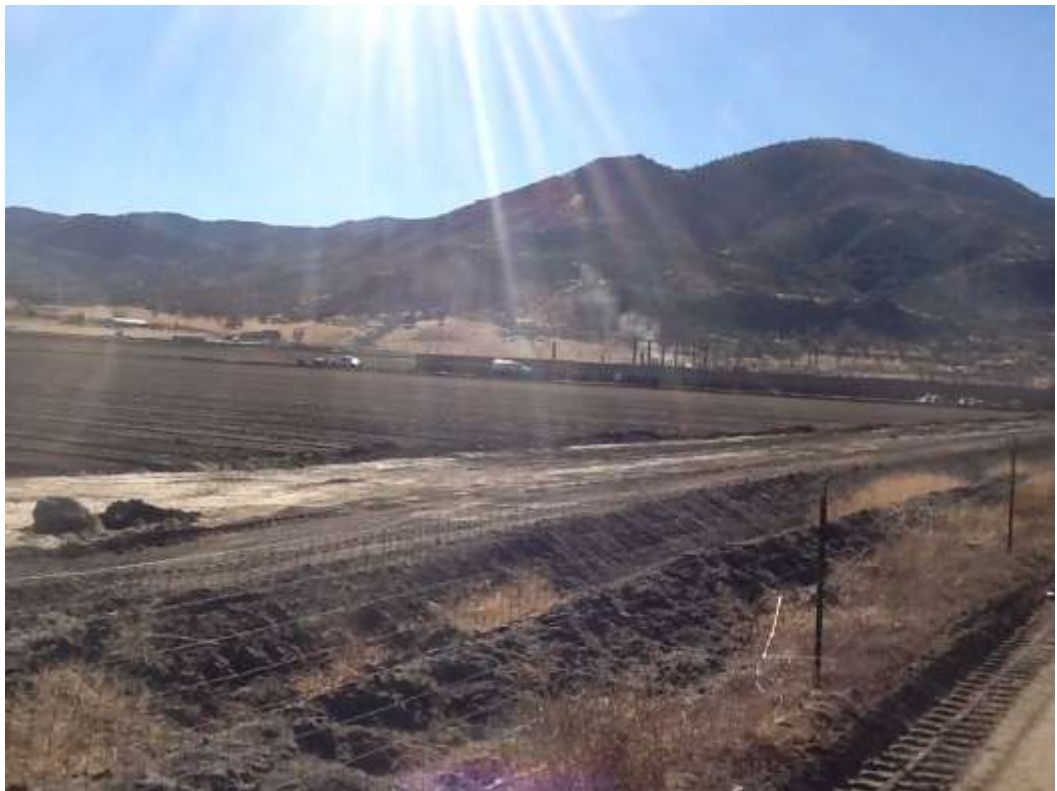
Figure 4 – Smoke coming from the Banducci Substation due to a malfunctioning cement pump.
