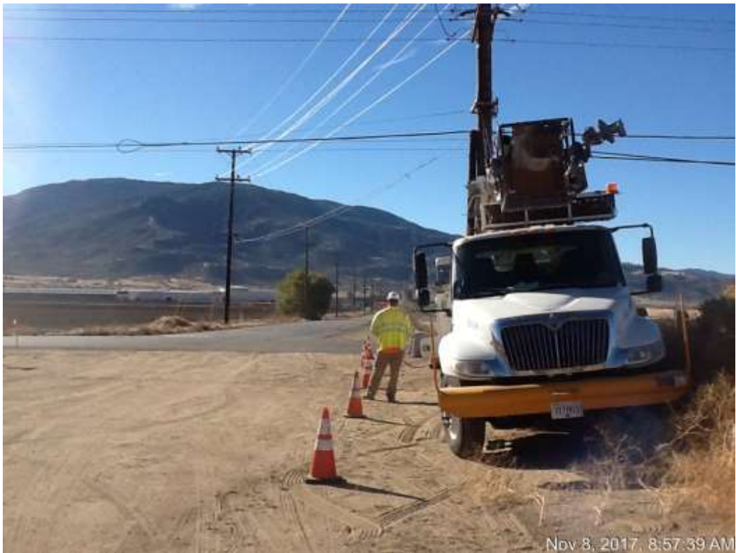
Figure 3 – Telecom crews installed fiber on Route 2 near the Banducci Substation.
