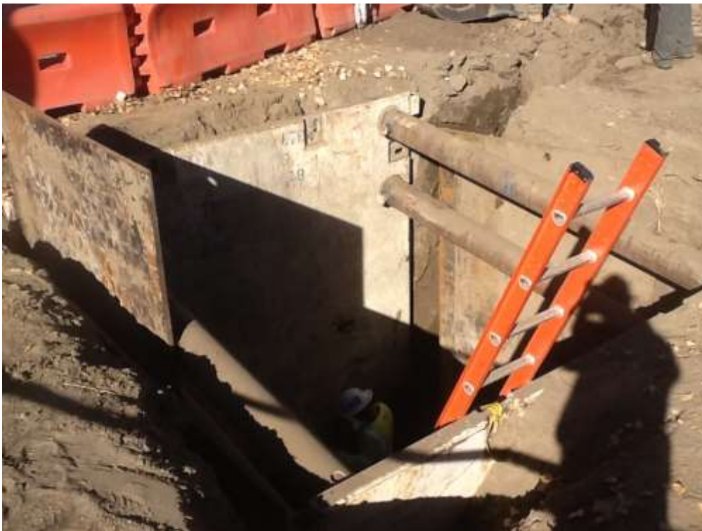
Figure 2 Trenching and vault tie in occurred along Pellisier Road.
