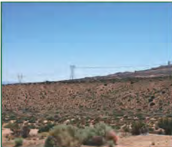
(Future Simulation) Looking east from Bowden Ranch Road in Arrastrae Canyon, Lucerne Valley. (Alternative, Segment 6)
