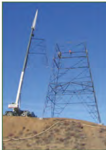
A crane carrying the top section of a LST for installation.
