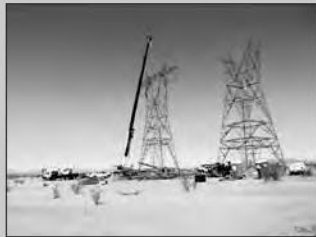
Ground-based Assembly
