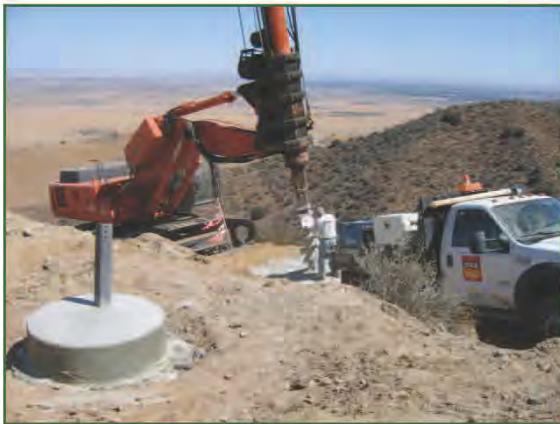
Foundation construction for an LST.
