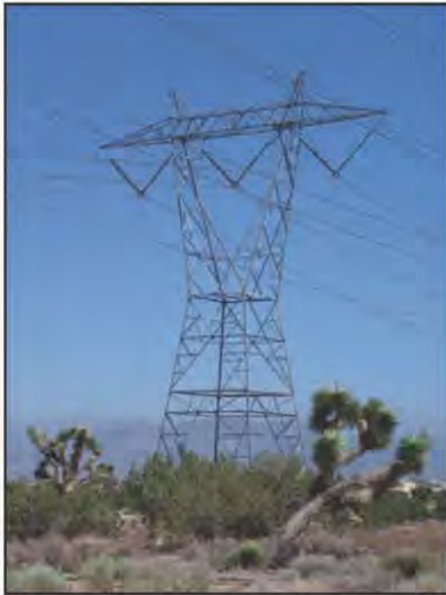
Example of a 500-kV single-circuit LST.
