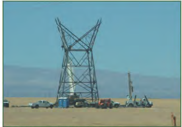
Transmission line tower construction site.
