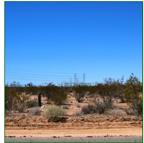
(Future Simulation) Desert View Substation facing west from Milpas Road, Apple Valley. (Proposed, Segment 5A)
