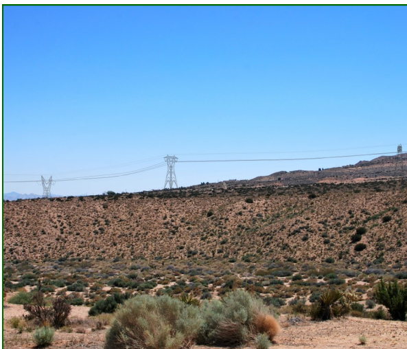
(Future Simulation) Looking east from Bowden Ranch Road in Arrastrae Canyon, Lucerne Valley. (Alternative, Segment 6)
