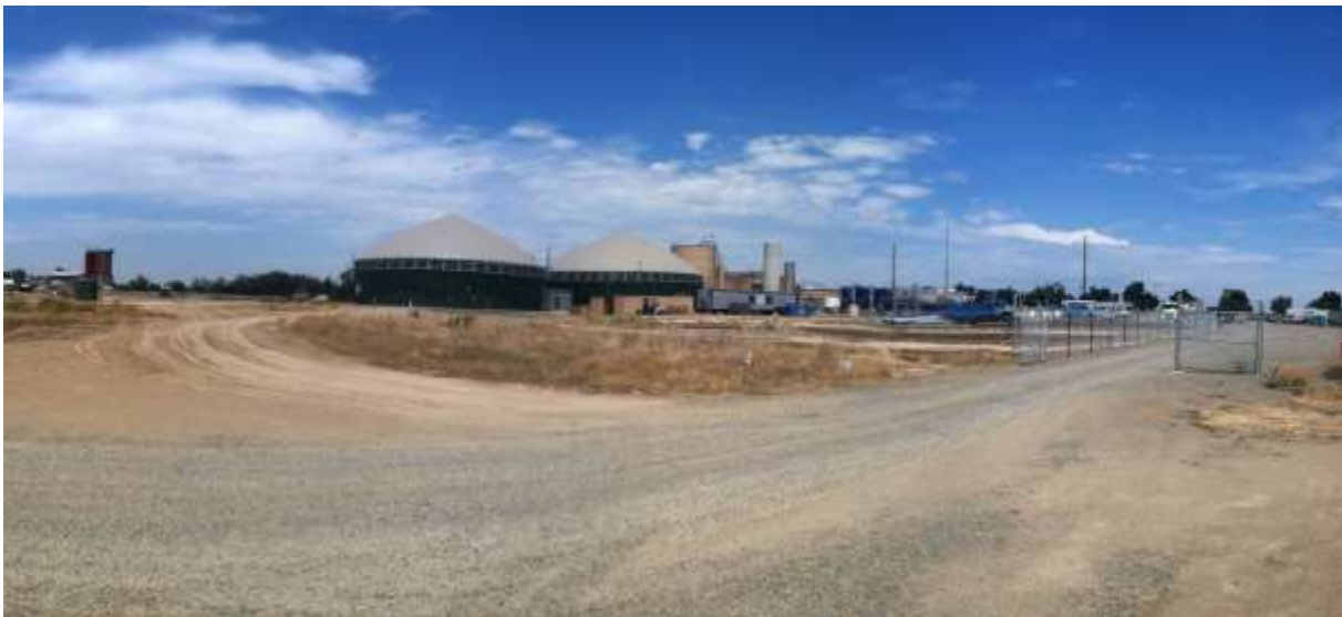
Figure 5 – Crews were redirected from using a dirt road to access between the Gallo substation and the Gallo staging area during the subject period. View northeast, 7/2/15.
