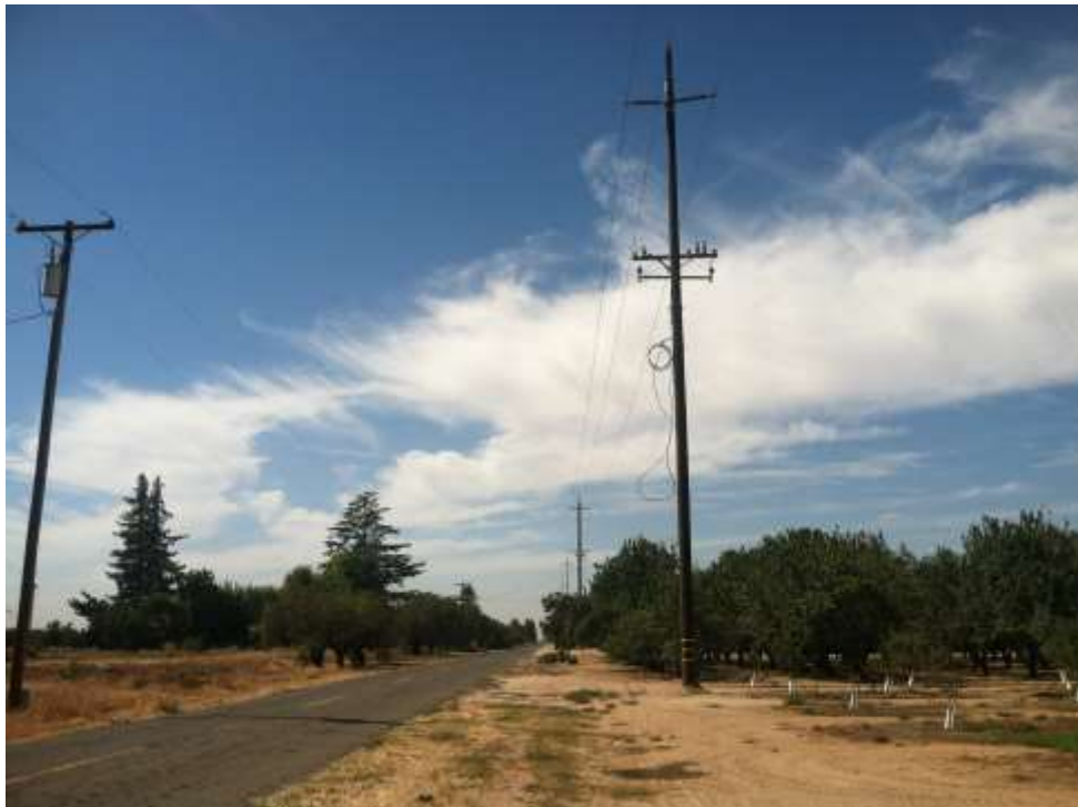
Figure 2 – Pole work in progress along Magnolia Avenue. View west 9/25/15.
