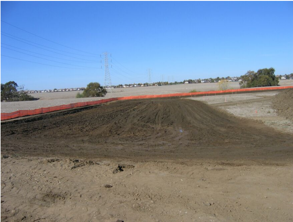
Figure 2 – Sub-grading at substation for berm construction, November 28, 2007.
