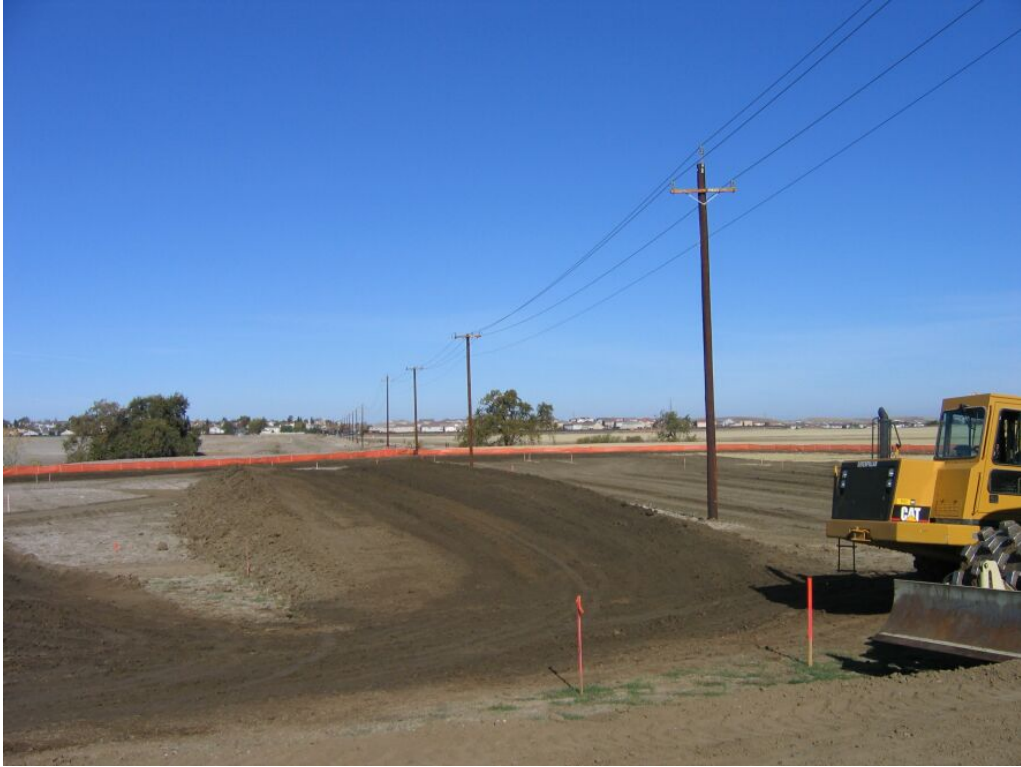
Figure 3 – Stockpiling of topsoil at substation, November 28, 2007.
