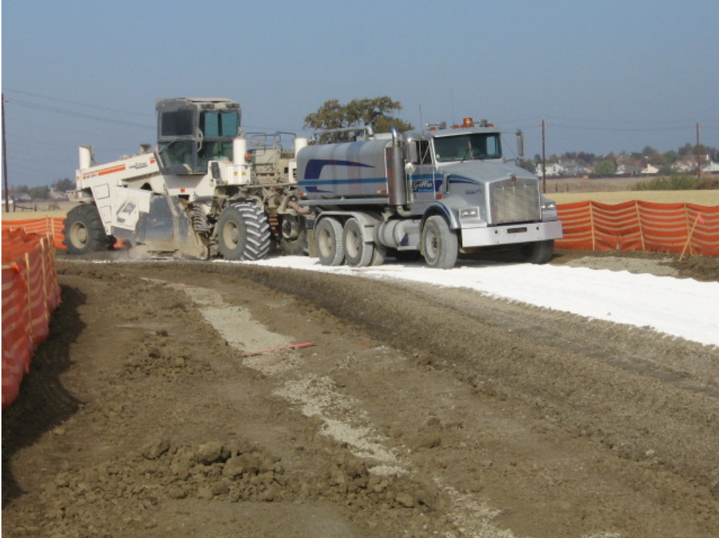
Figure 1 – Lime treating of access road, November 28, 2007.
