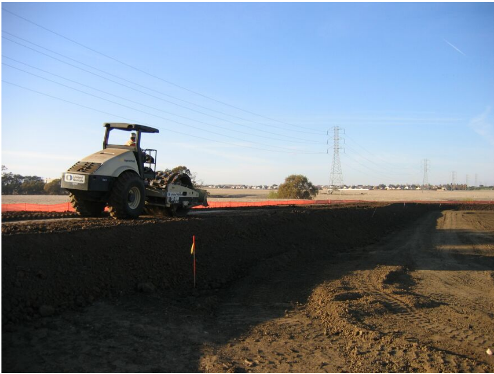
Figure 3 – Berm on west side of substation being created, December 5, 2007.
