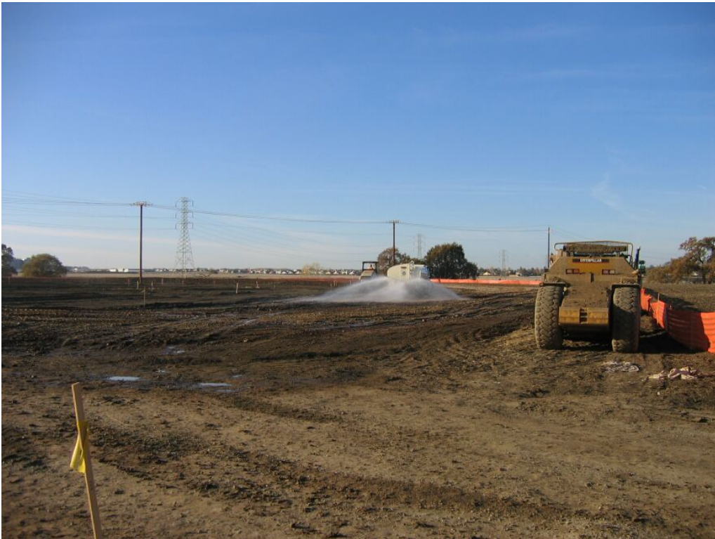
Figure 2 – Sub-grading and compacting at substation site, December 5, 2007.
