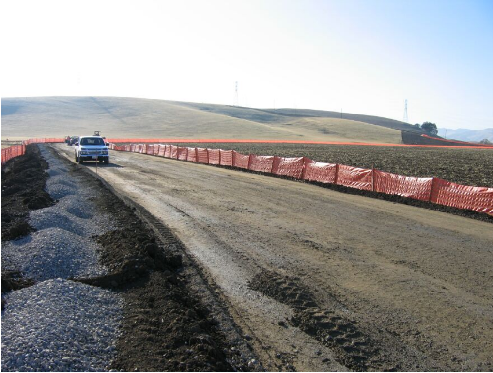
Figure 1 – Access road to substation with wildlife exclusion fencing installed, December 5, 2007.
