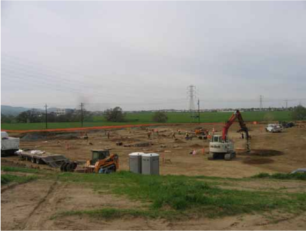
Figure 1 – Crews starting foundation work at substation site, March 7, 2008.
