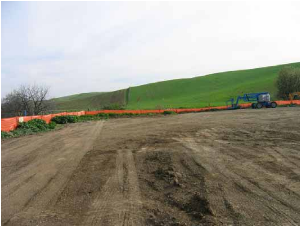
Figure 4 – Staging yard/laydown yard on the north side of Sand Creek, March 7, 2008.
