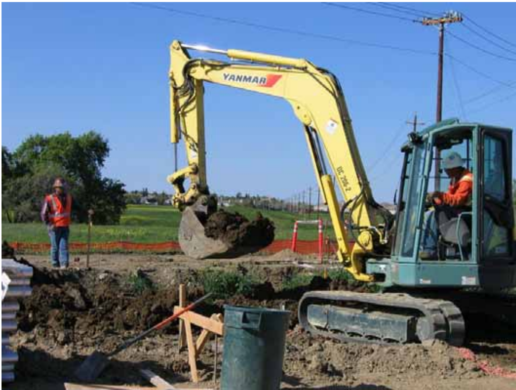
Figure 4 – Crews starting excavation of SPCC pond, March 27, 2008.
