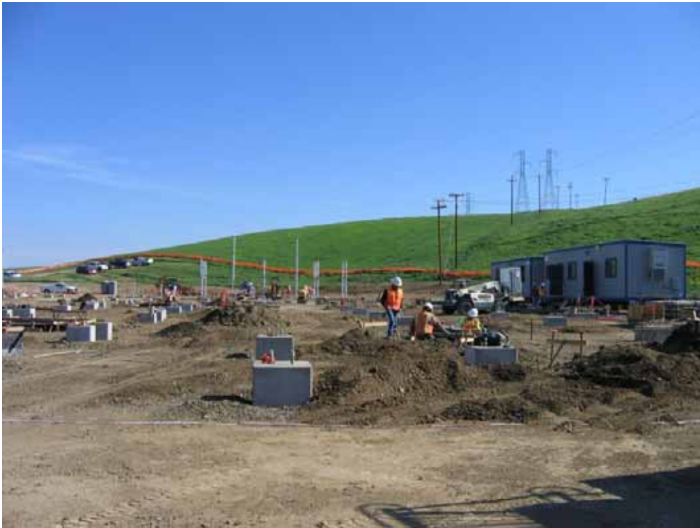
Figure 3 – Crews working on foundations at the substation site, March 27, 2008.
