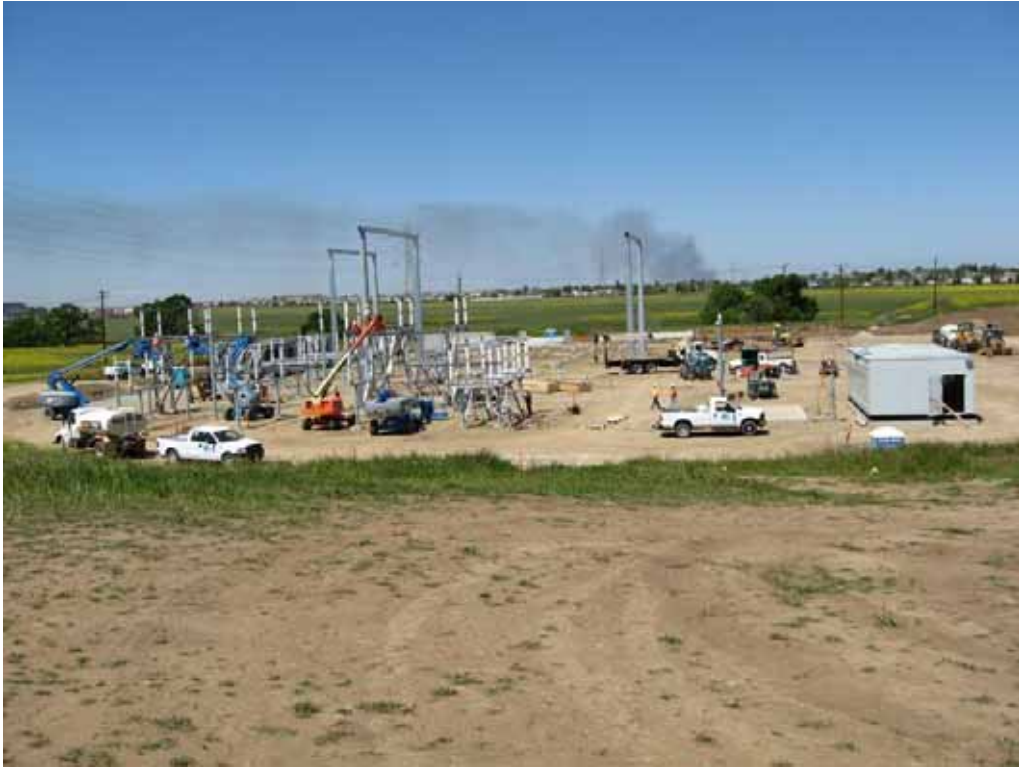
Figure 1 – View of substation site looking north, April 11, 2008. (Photo courtesy of TRC)
