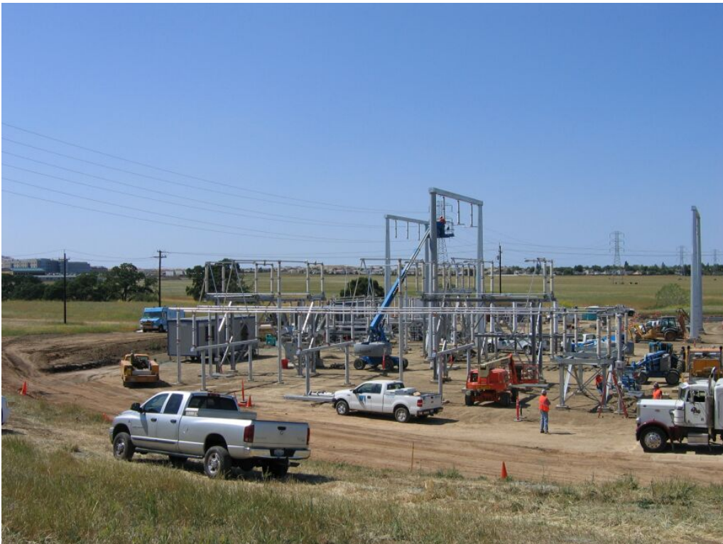
Figure 2 – View of substation site looking northwest, April 30, 2008.
