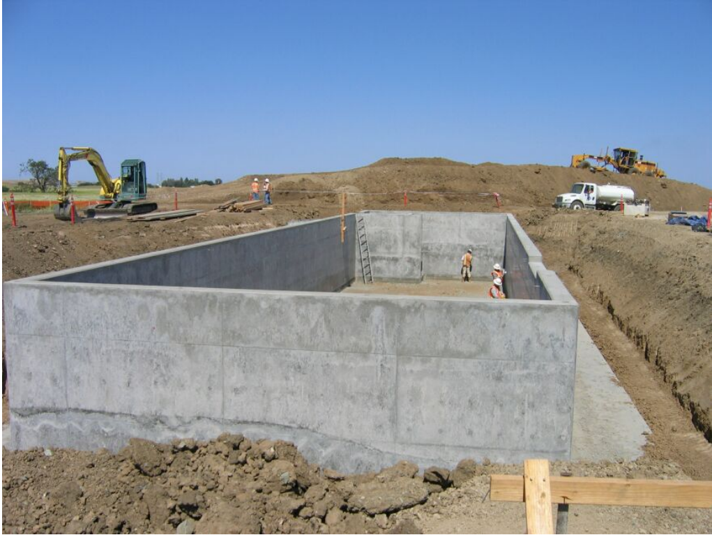
Figure 5 – Crews working on the SPCC pond, April 30, 2008.
