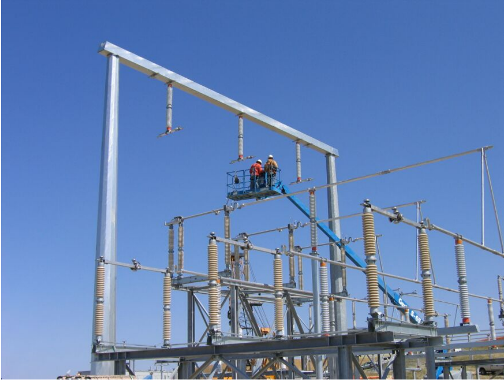
Figure 1 – Crews working on buswork structures, April 30, 2008.
