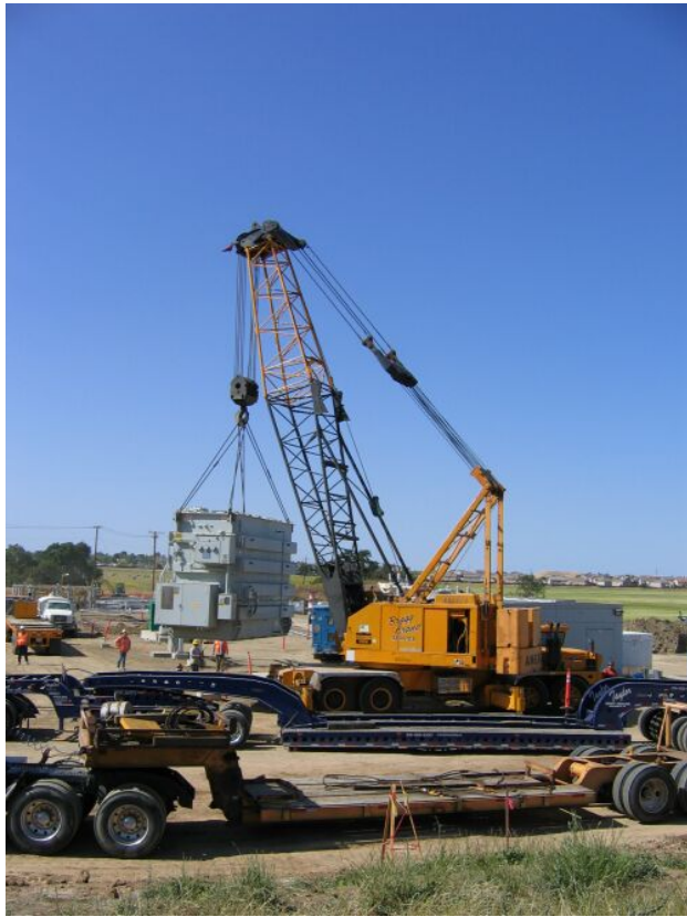
Figure 3 – Crane installing transformer on foundation, April 30, 2008.
