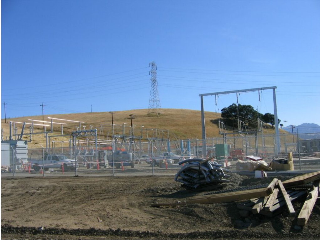
Figure 3 – Substation site with security fence installed around the outside, May 16, 2008.
