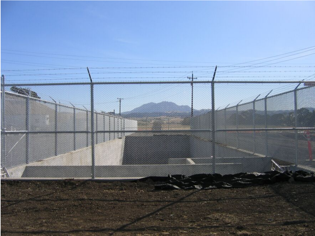
Figure 2 – SPCC Pond with security fencing installed around the outside, May 16, 2008.
