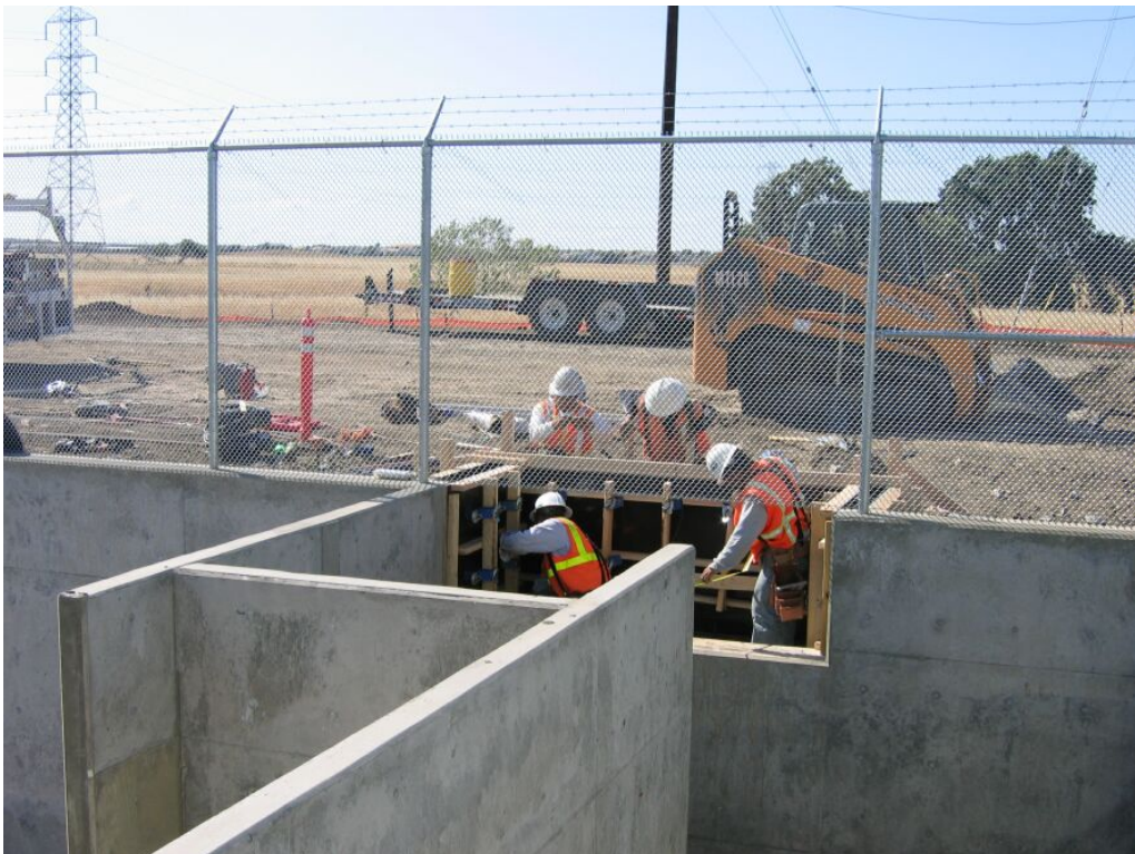
Figure 4 – Crews working on SPCC pond, May 29, 2008.
