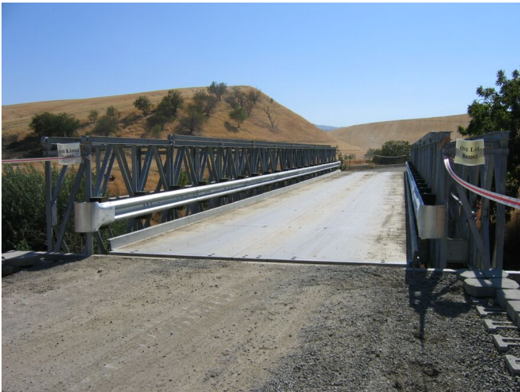
Figure 4 – New guard rail installed on bridge over Sand Creek, September 18, 2008.
