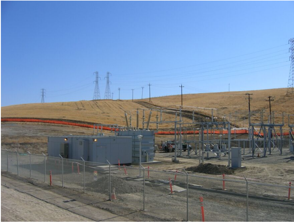
Figure 1 – View of the substation site looking southwest, September 18, 2008.
