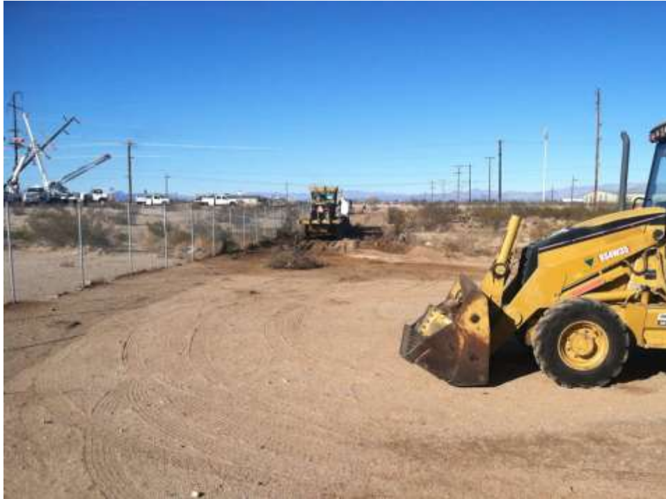
Figure 1 – Grubbing and grading occurred. View north, November 17, 2014.
