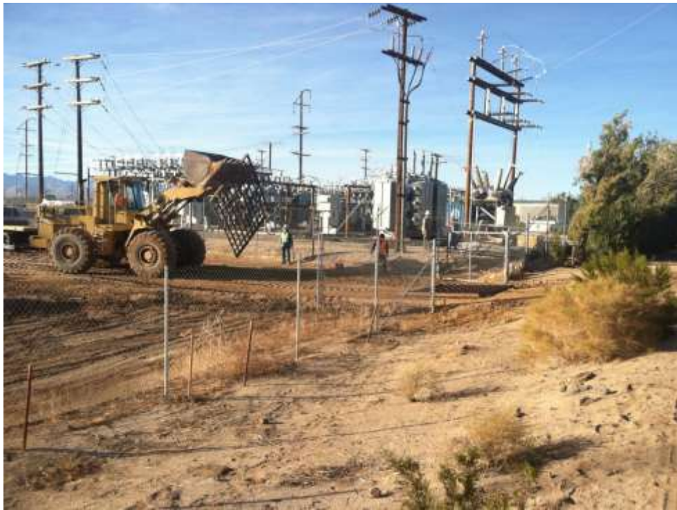
Figure 3 – Rumble strip placement at site entrance. View northwest, November 17, 2014.
