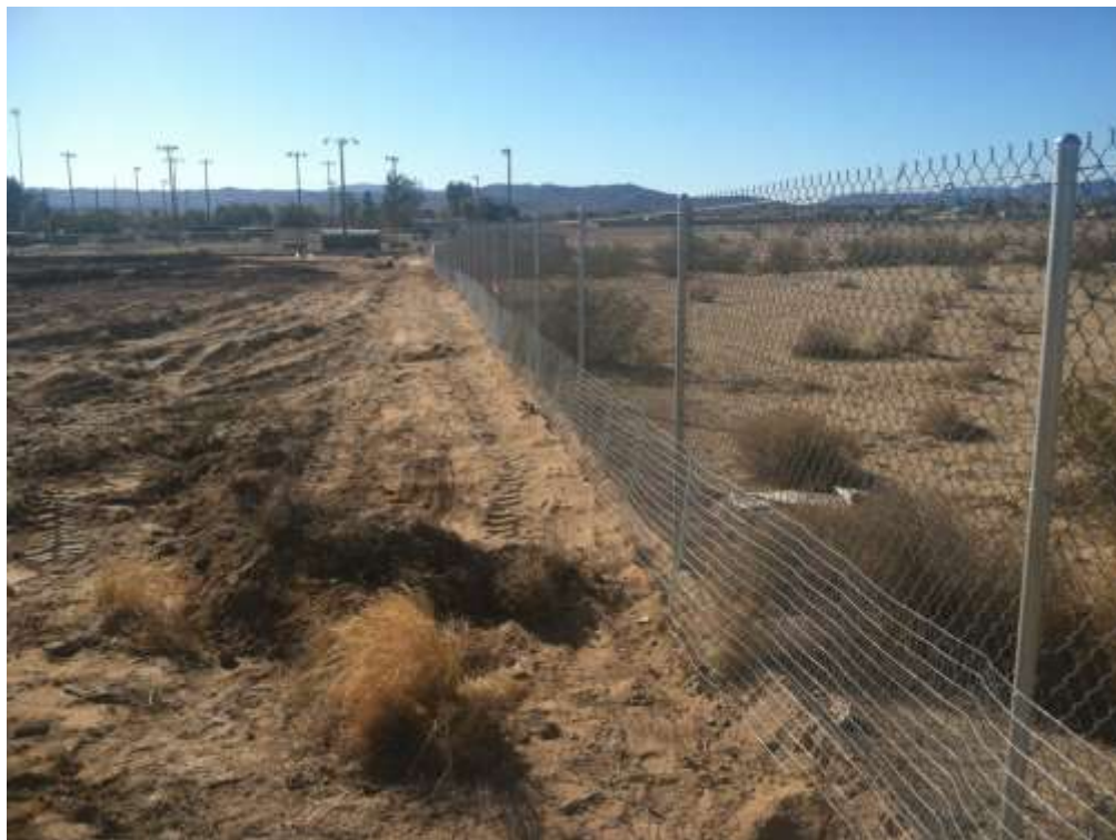
Figure 4 –Temporary tortoise fence installed along work limits. View south, November 21, 2014.
