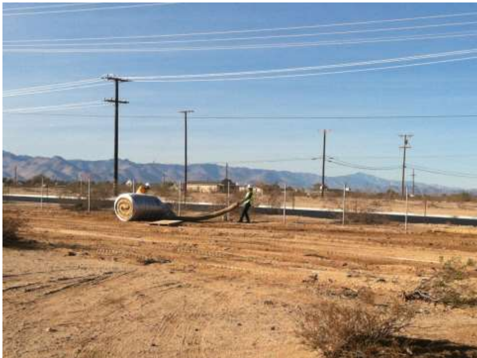
Figure 2 – BMP (fiber roll) installation. View northwest, November 17 2014.
