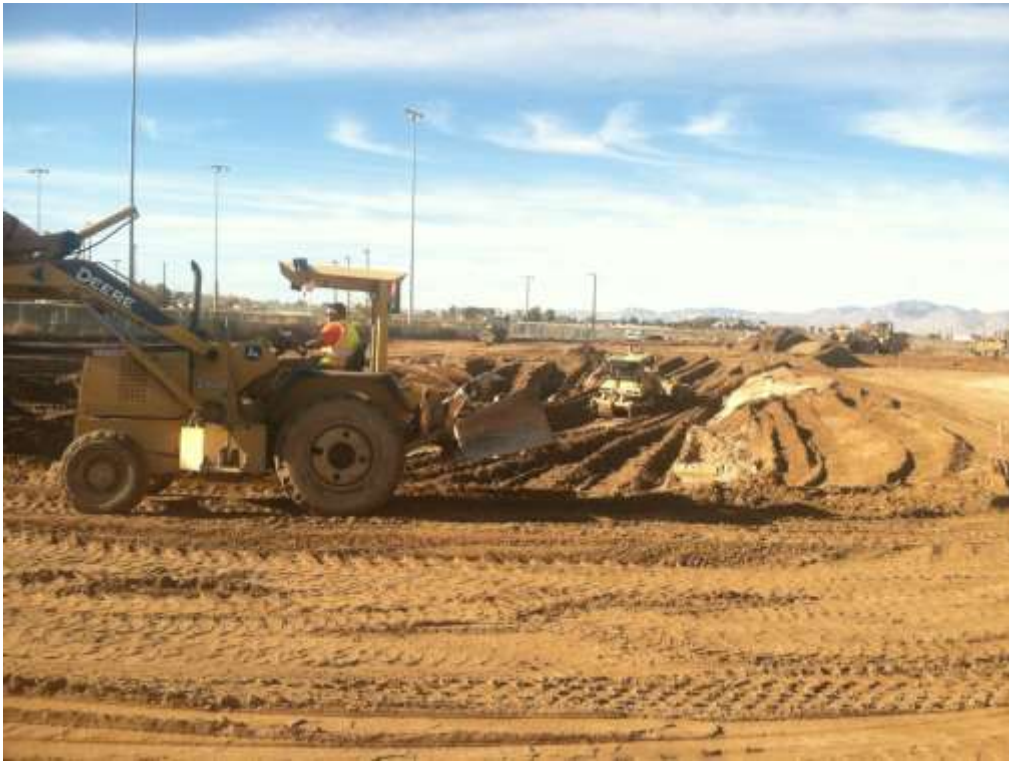
Figure 1 – Grading continued. View west, December 9, 2014.
