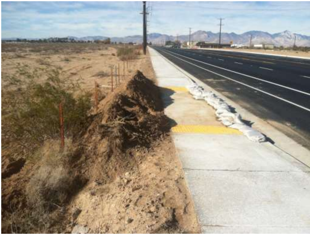
Figure 8 –Soil pile was placed at a stormwater outlet, along Ridgecrest Boulevard. View west, December 9, 2014.
