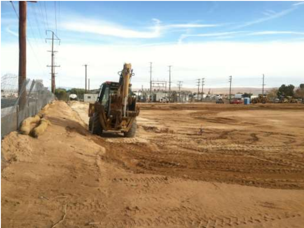
Figure 1 – Grading continued. View east, December 15, 2014.
