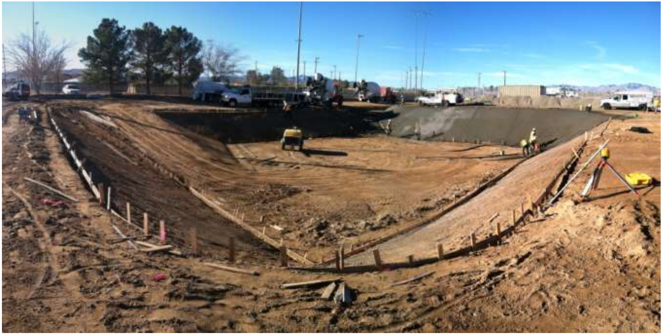
Figure 6 – Installation of the detention basin. View southwest, January 8, 2015.
