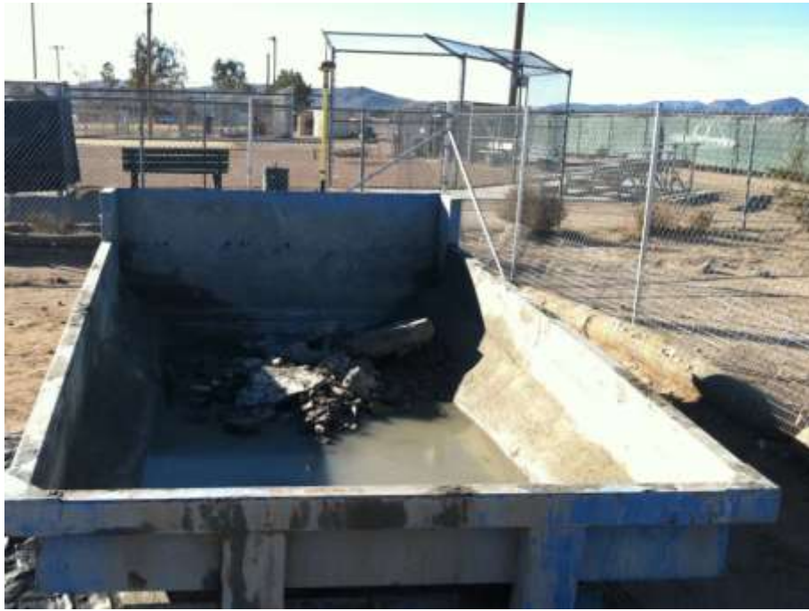
Figure 8 – Concrete wash is adequately contained. View south, January 8, 2015.
