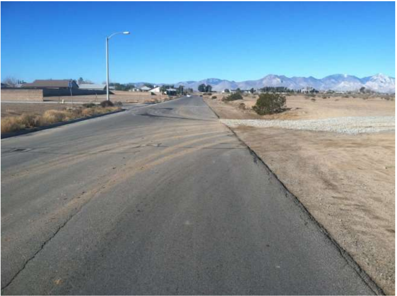
Figure 8 – Recent rains and mud generated some track out onto Church Avenue. View west, January 13, 2015.
