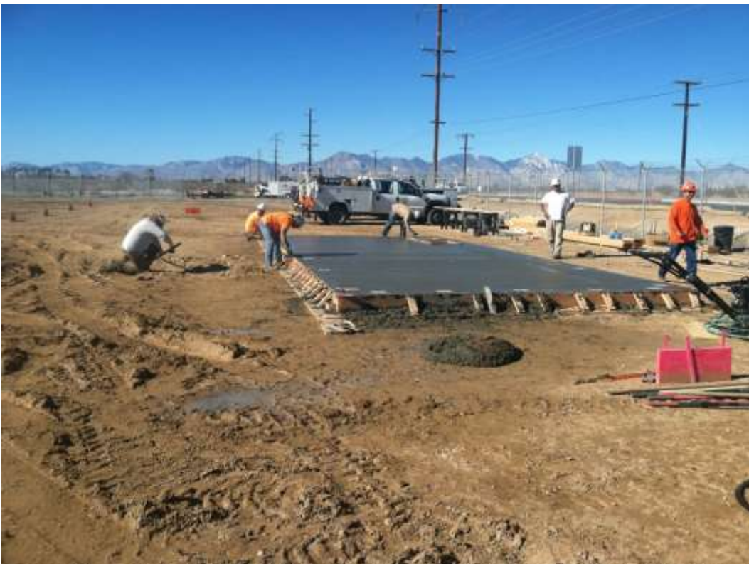
Figure 4 – Pouring of concrete for the MEER building occurred. View west, January 13, 2015.
