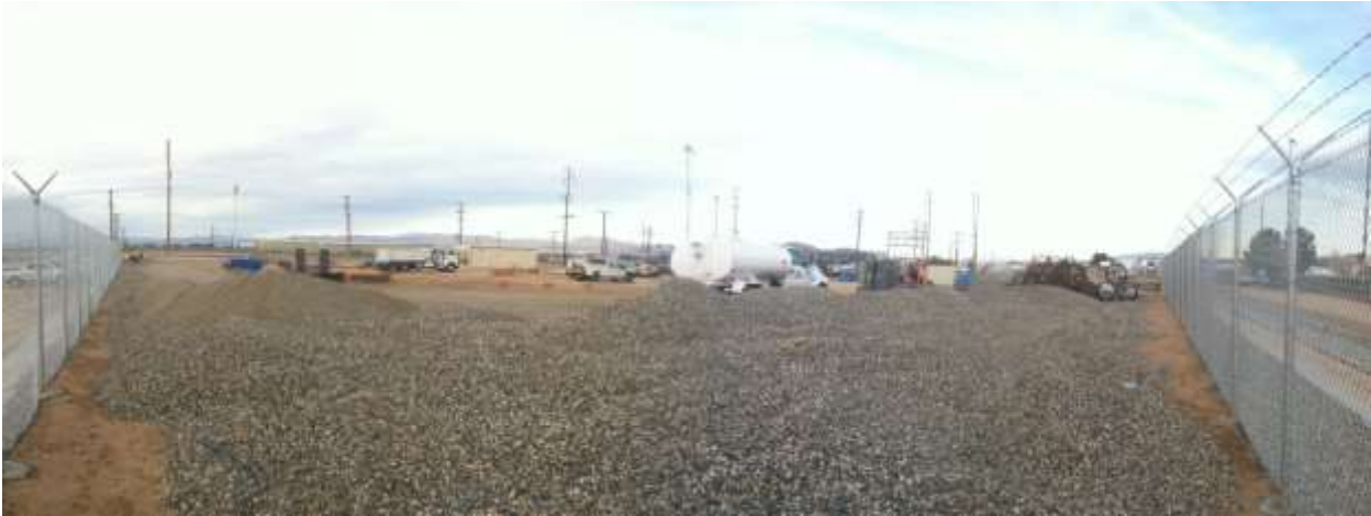
Figure 1 – Gravel continues to be stored on the substation pad. View northeast, January 22, 2015.
