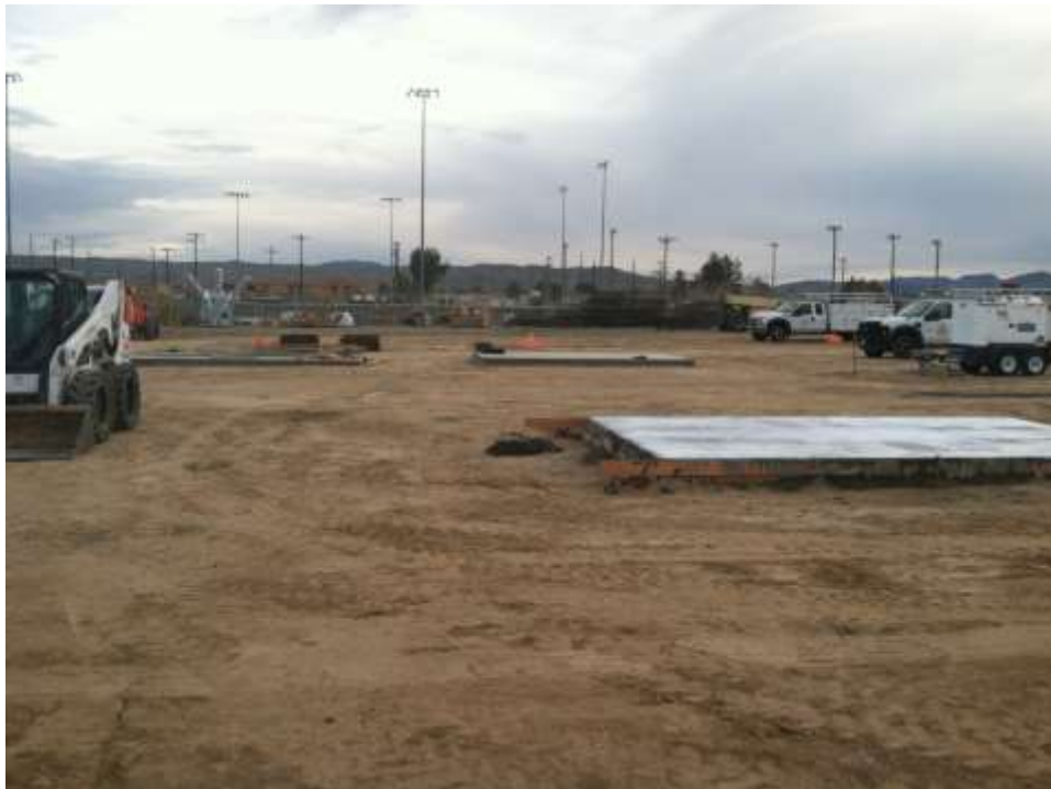
Figure 2 – Foundations were installed during the subject period. View south, January 22, 2015.
