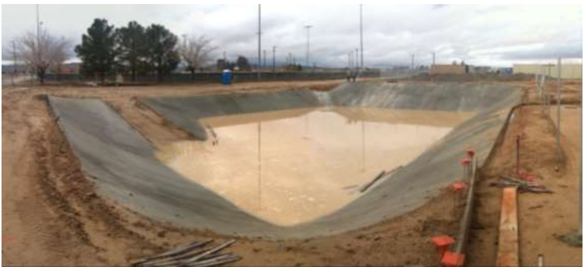
Figure 3 – Pooled water has slowed completion of the site's detention basin. View southwest 01/08/15 above, 01/13/15 middle, 01/27/15 below.
