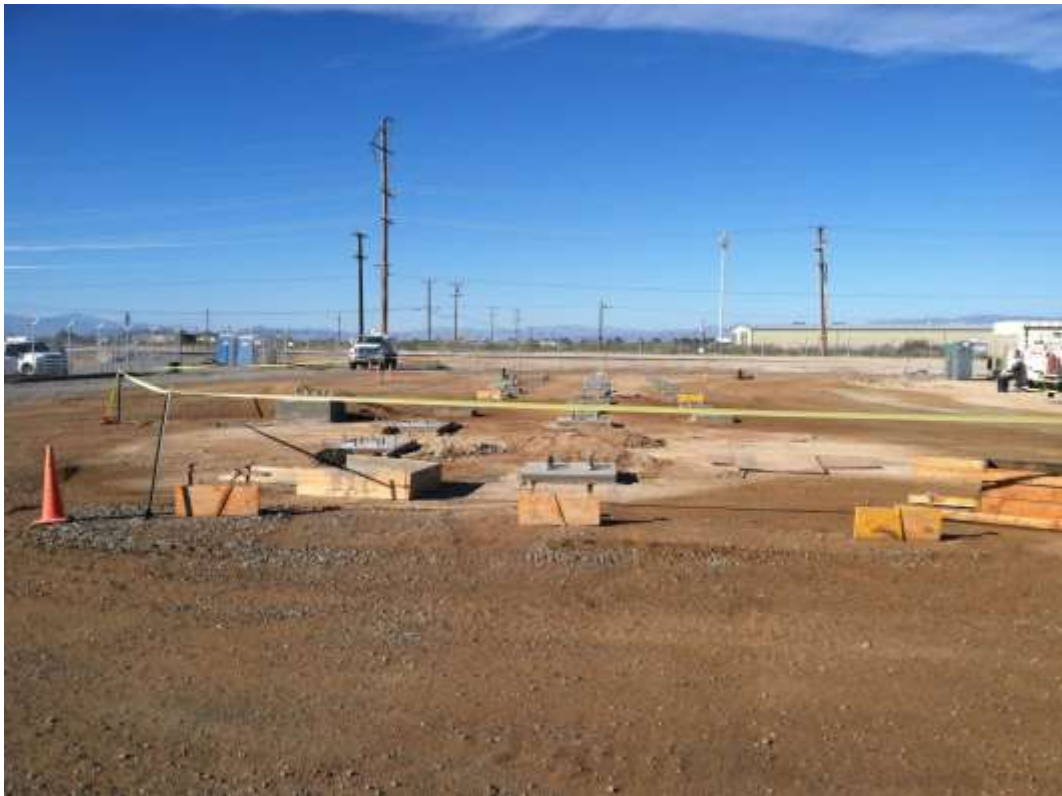
Figure 2 – Foundation installation continues in the substation expansion area. View north, 02/19/15.
