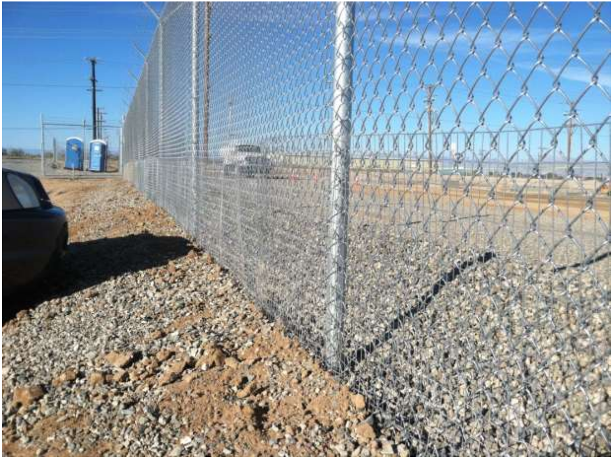
Figure 4 – Installation of additional desert tortoise fencing occurred. View north, 02/19/15.
