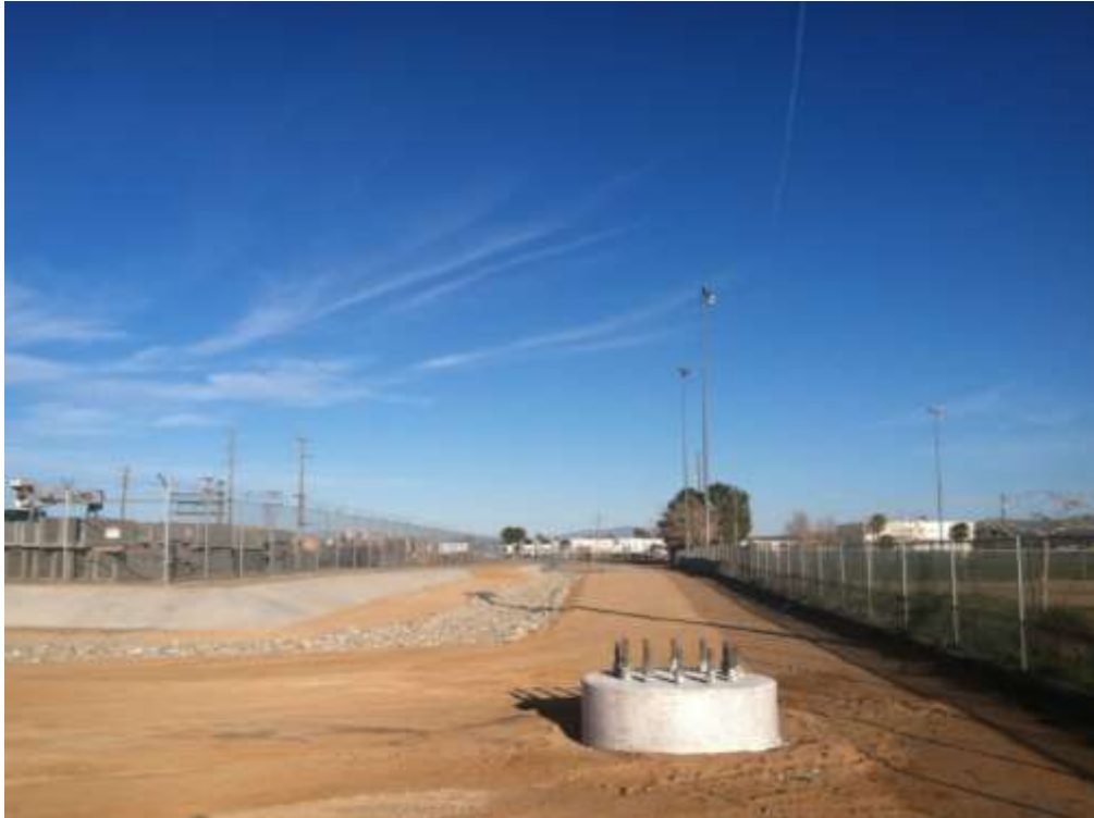
Figure 1 – Foundations for TSPs were installed during the subject period. View east, 02/26/15.
