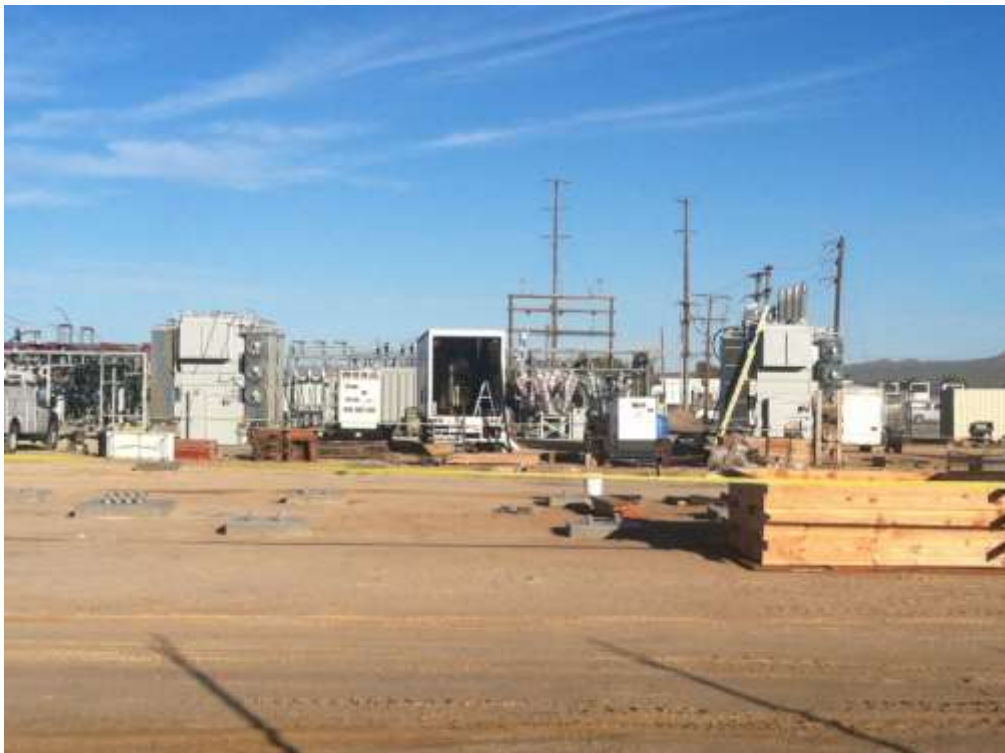
Figure 2 – Two new transformers were installed during the subject period. View east, 02/26/15.
