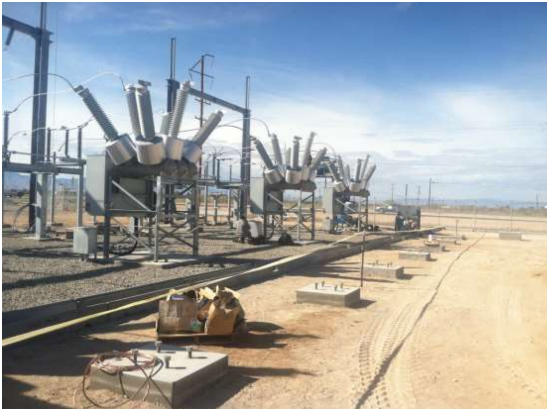
Figure 2 – Structure installation occurred during the subject period. View northwest, 03/24/15.
