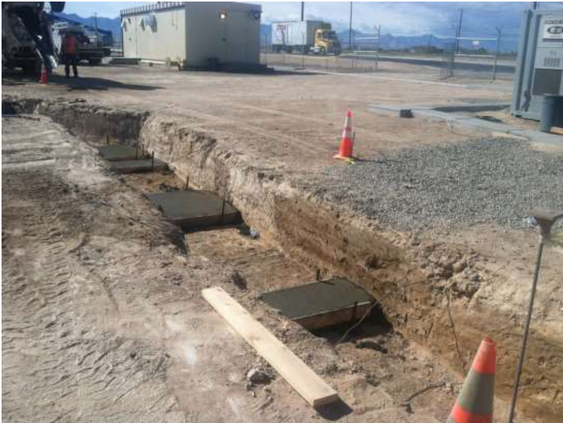
Figure 4 – Trenching continues at Downs Substation. View northwest, 03/24/15.
