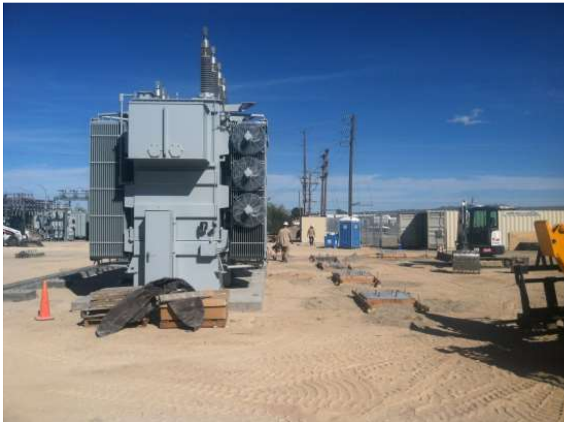
Figure 3 – Foundation installation continues at Downs Substation. View east, 03/24/15.
