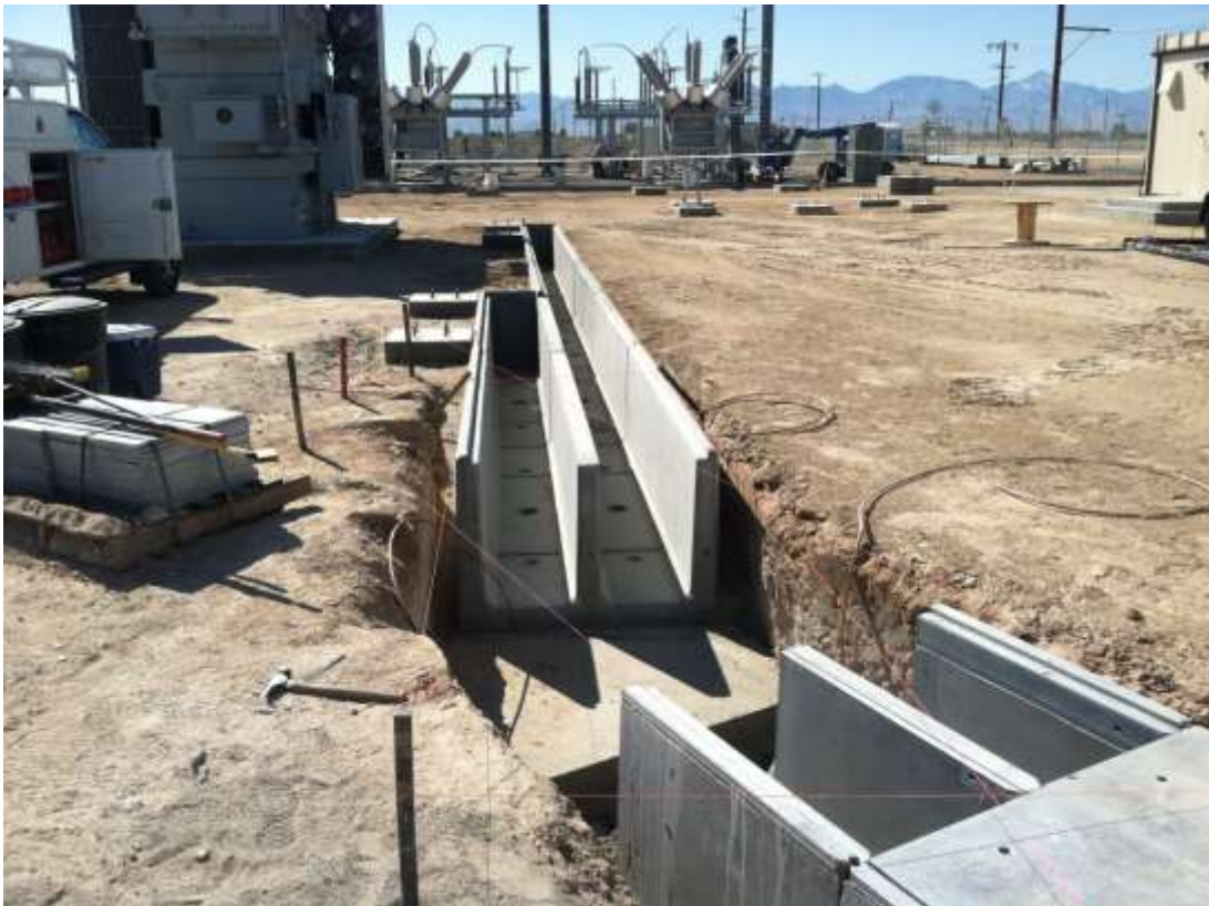
Figure 3 – Trenching continues at Downs Substation. View west, 03/30/15.
