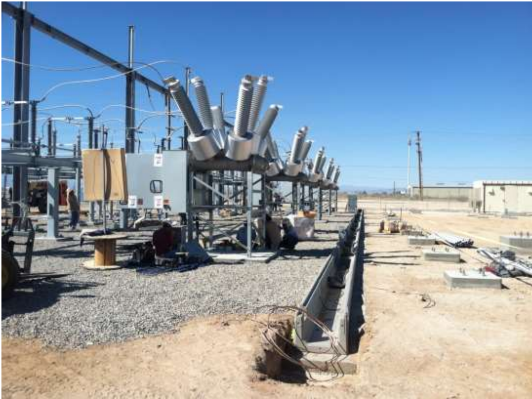
Figure 2 – Structure installation occurred during the subject period. View northwest, 03/30/15.
