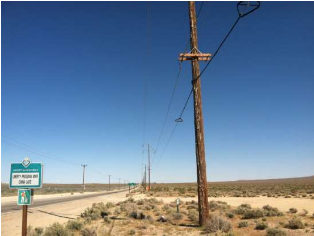
Figure 6 – A recently installed section of telecom line (attached to horizontal wood supports) is seen at the corner of Ridgecrest Boulevard and San Bernardino Boulevard. View east, 03/30/15.
