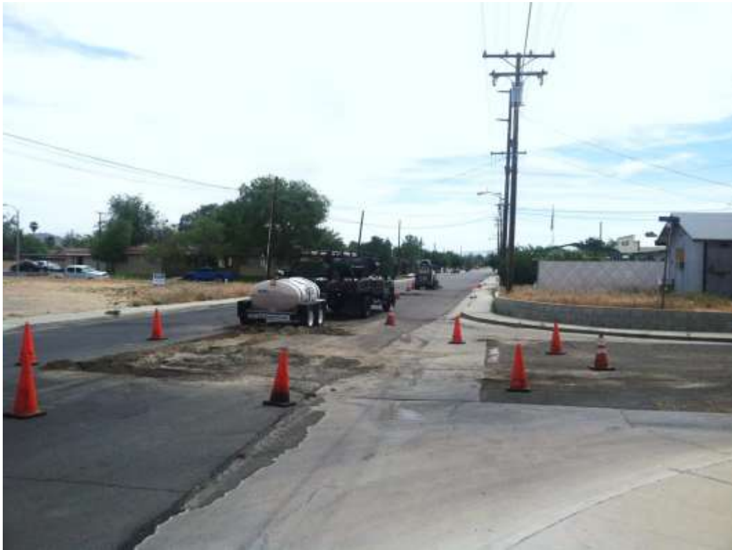
Figure 4 – Roadway repair work occurred along the underground telecom route. View east, 4/30/15.
