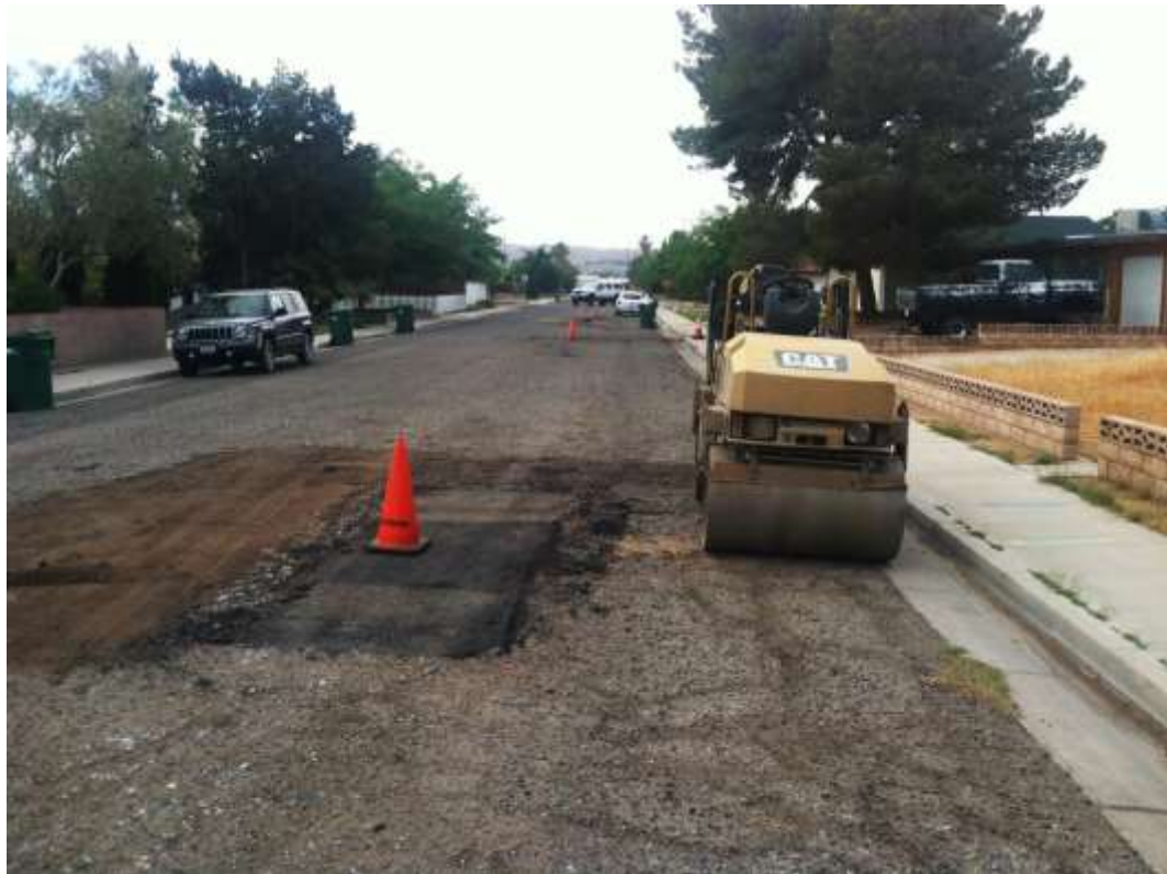
Figure 5 – Roadway repair work occurred along the underground telecom route. View south, 4/30/15.
