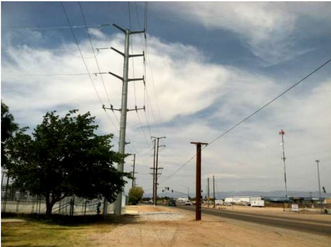
Figure 3 – TSP installation is complete at Downs Substation. View north, 05/11/15.
