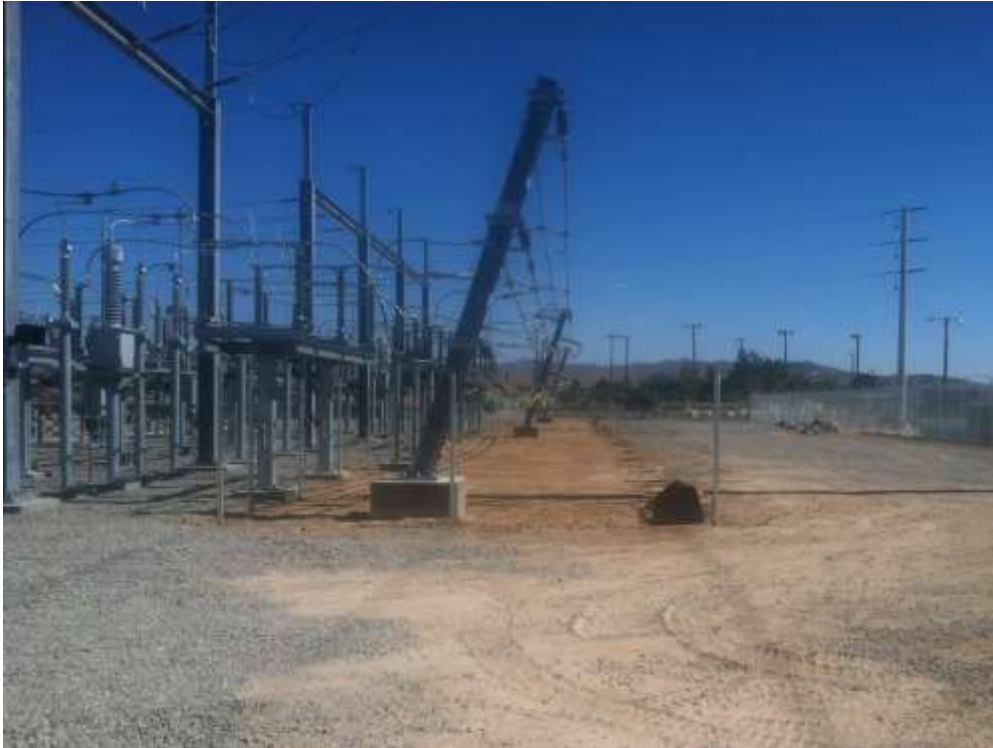
Figure 1 – Installation of interior fencing occurred during the subject period. View south, 6/16/15.
