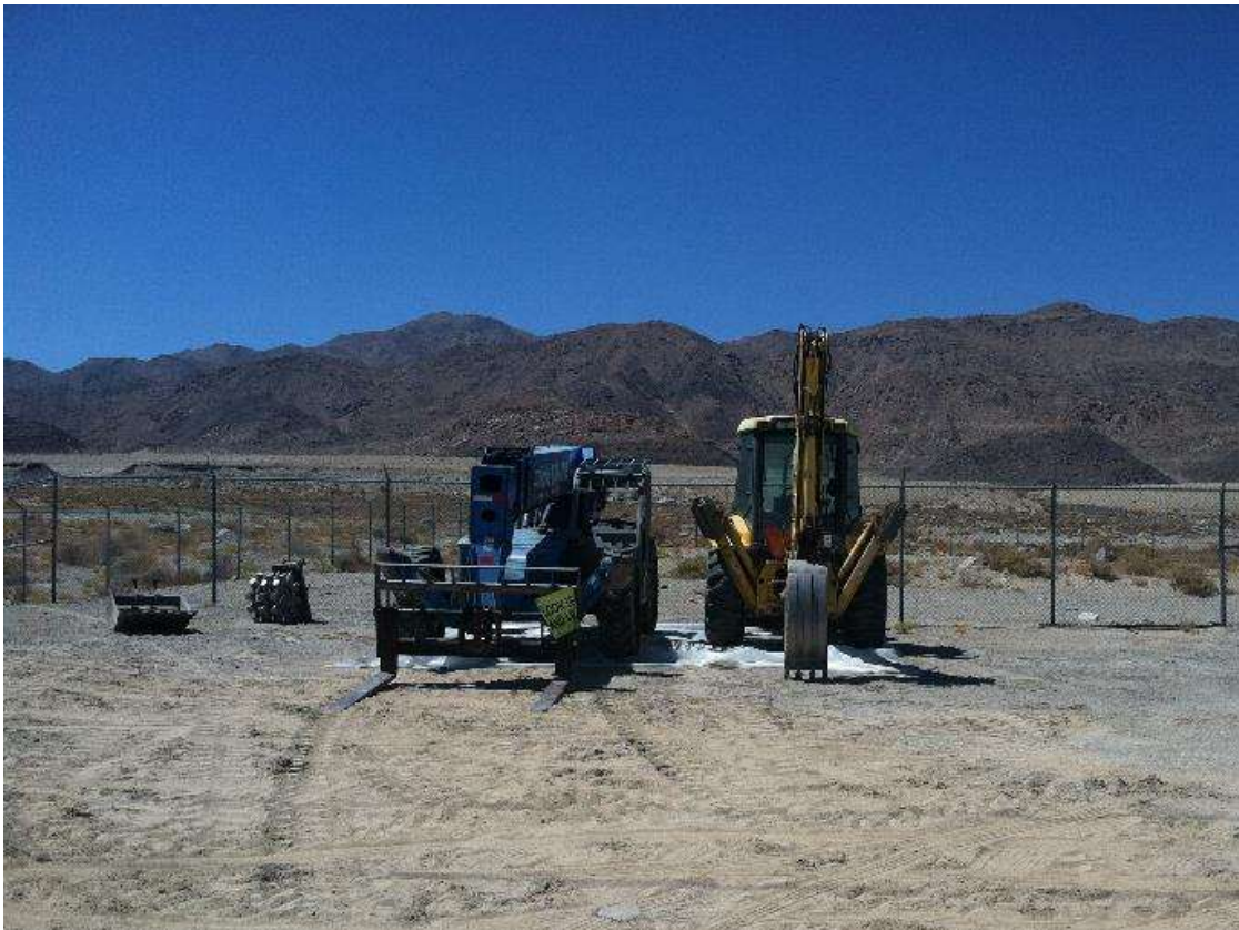
Figure 3 – Equipment used secondary containment during the subject period. View northwest, 7/16/2015.
