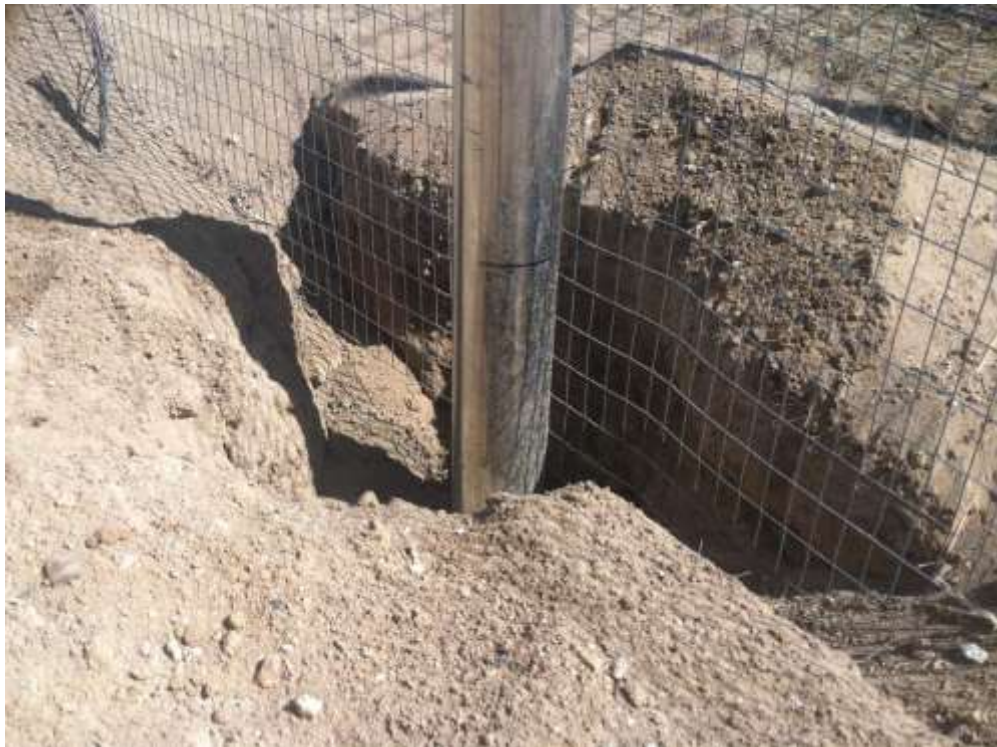
Figure 2 – Desert tortoise proof fencing was installed along the Downs Substation perimeter fence. View southeast.
