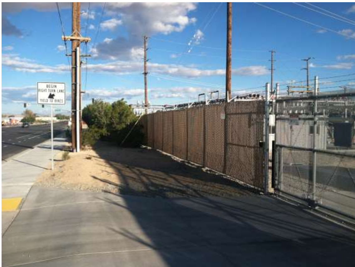
Figure 2 – Fence crews completed the perimeter fencing at Downs Substation during the subject period. View east (10/5/15 above, 10/20/15 below).
