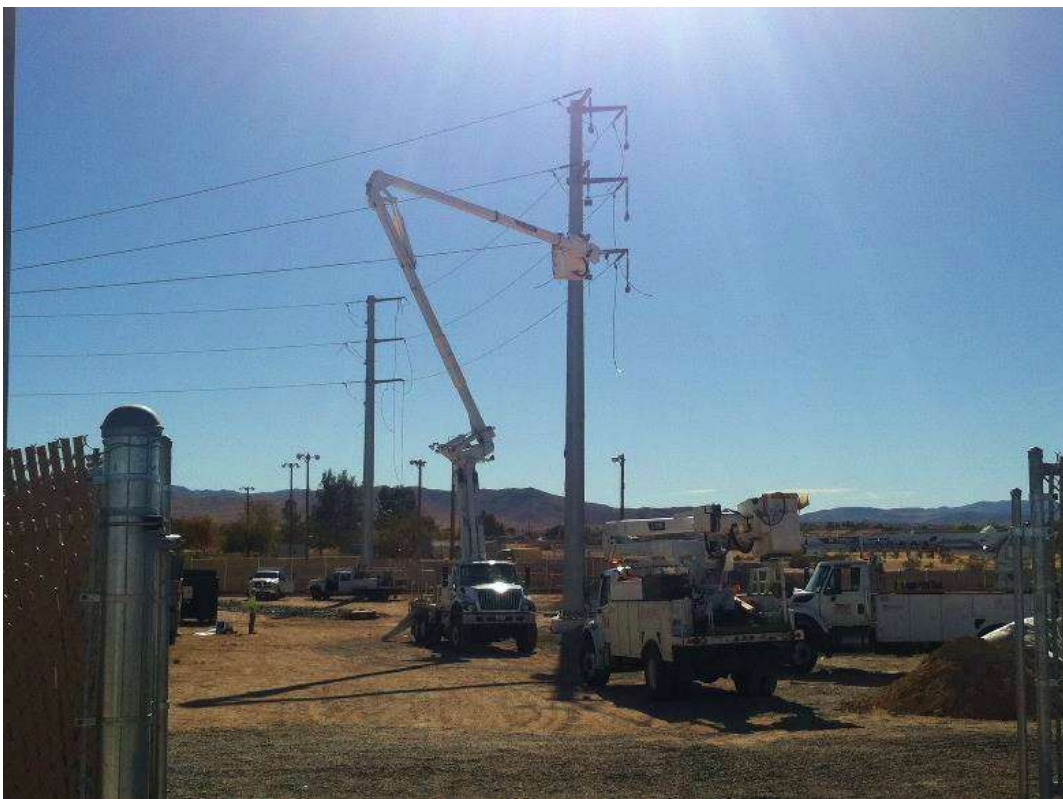
Figure 2 – Crews installed a TSP during the subject period. View south (11/20/15).
