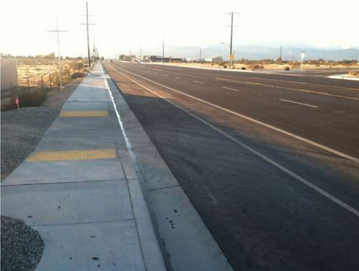
Figure 3 – Roadway entrances are swept to remove track out. View west (11/25/15).
