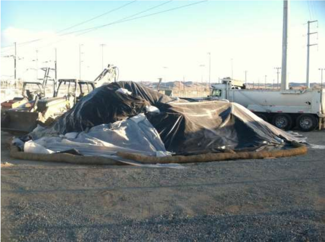
Figure 3 – SWPPP BMPs were in place during the subject period. View south 12/14/15.
