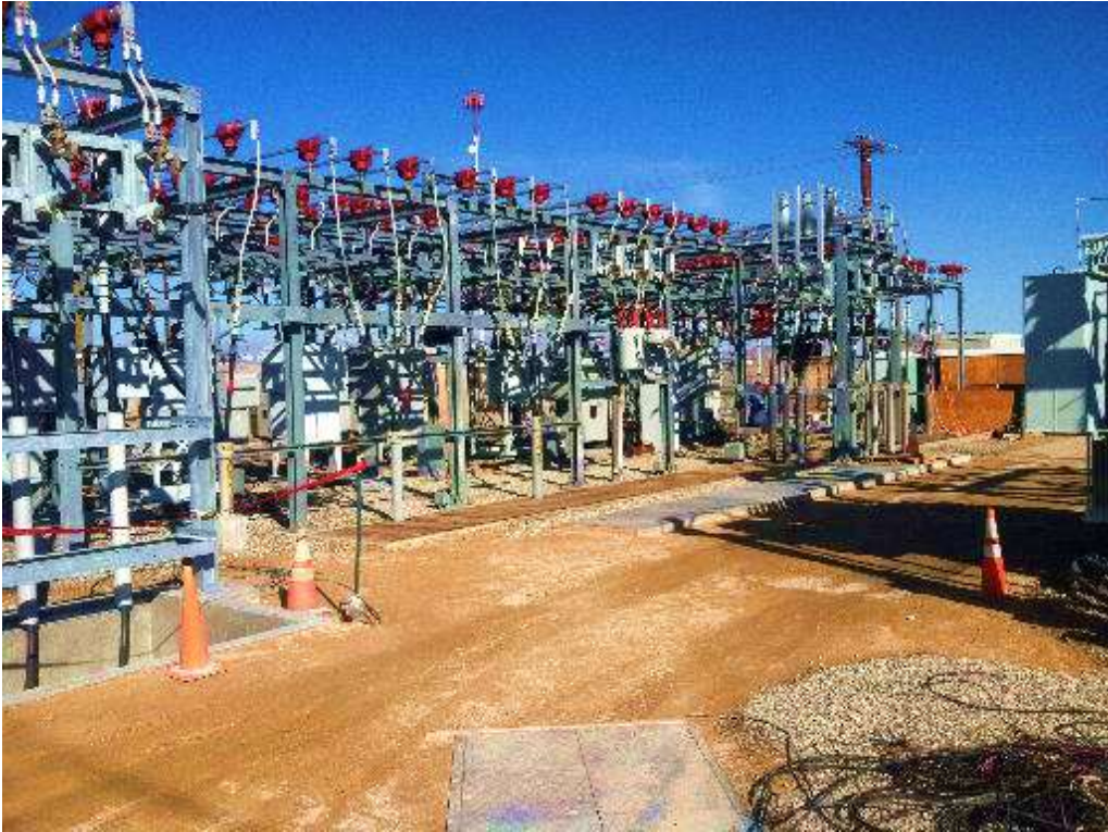
Figure 1 – Crews were upgrading existing structures during the subject period. View northeast, 1/20/16.
