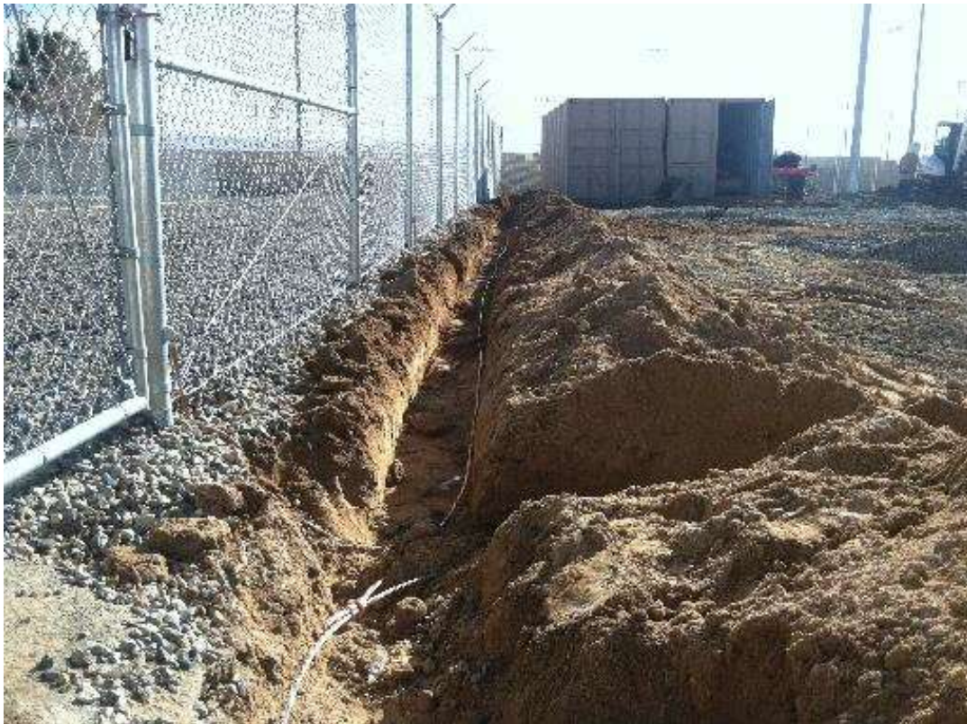
Figure 4 – Grounding cable installation was completed during the subject period. View south 01/20/16.
