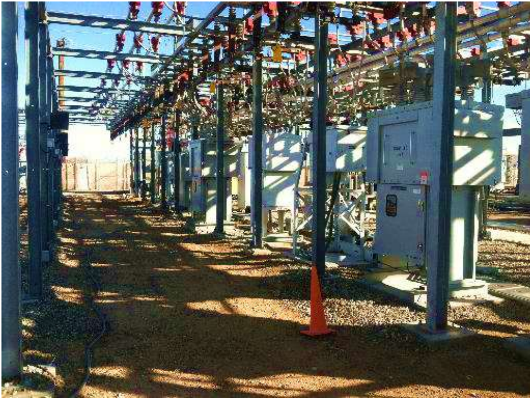
Figure 3 – Old equipment to be remove. View east 01/20/16.
