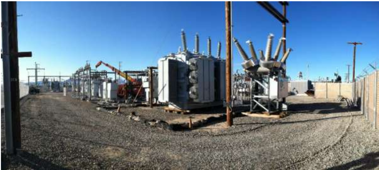
Figure 3 – Crews dismantle old 33 kV structures during the subject period. View northwest 01/25/16.
