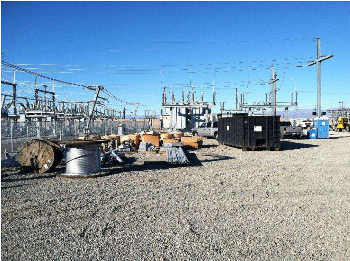
Figure 4 – Equipment and materials remain stored onsite. View north 01/25/16.
