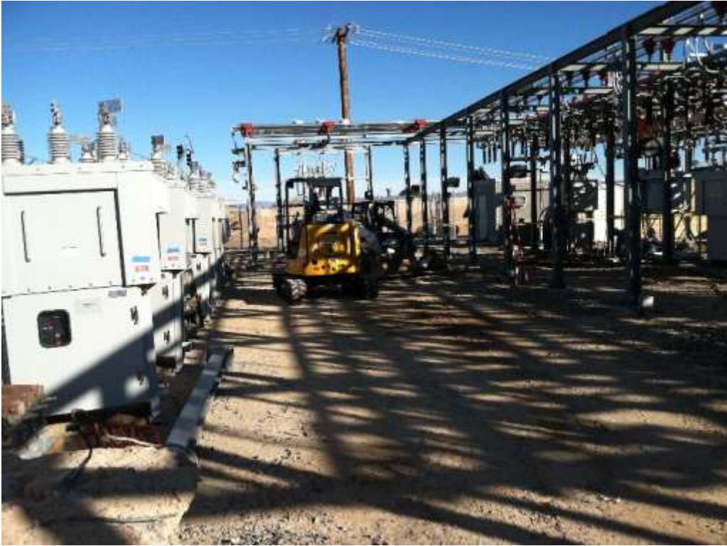
Figure 1 – Crews were upgrading existing structures during the subject period. View east, 1/25/16.
