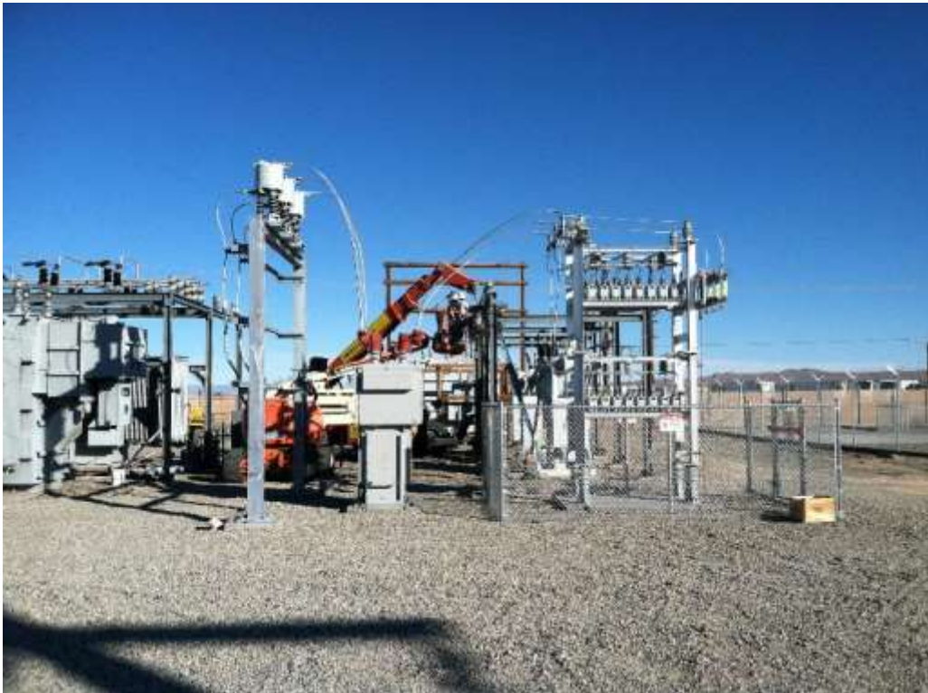
Figure 2 – Crews dismantle old 33 kV structures during the subject period. View east 01/25/16.
