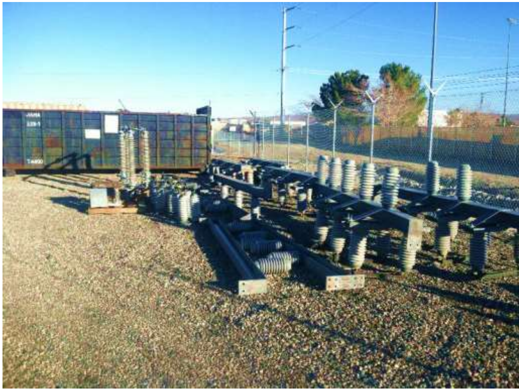
Figure 4 – Equipment and materials remain stored onsite. View east 02/02/16.
