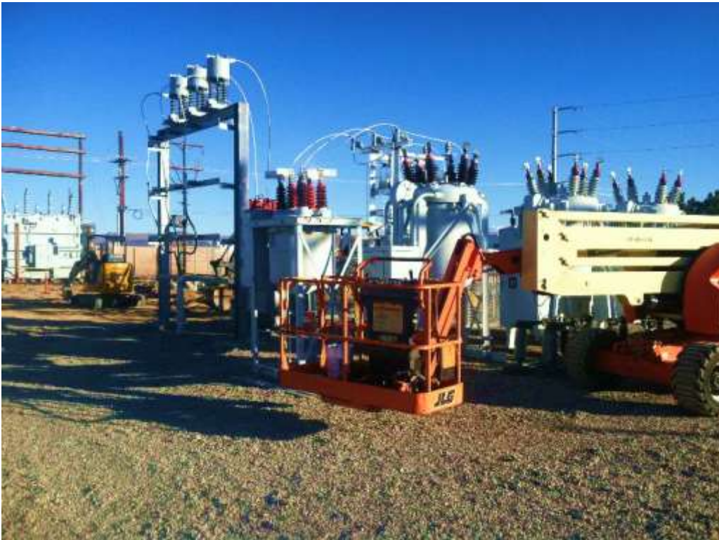
Figure 2 – Crews dismantle old 33 kV structures during the subject period. View east 02/02/16.
