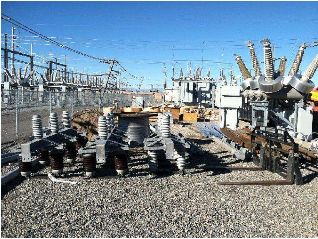
Figure 4 – Equipment and materials remain stored onsite. View north 02/08/16.
