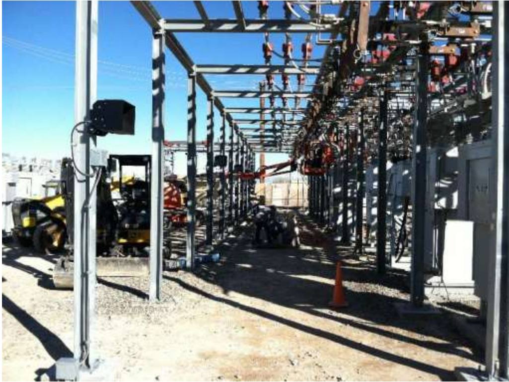
Figure 1 – Crews continued installing replacing breakers and installing foundations. View east, 02/08/16.
