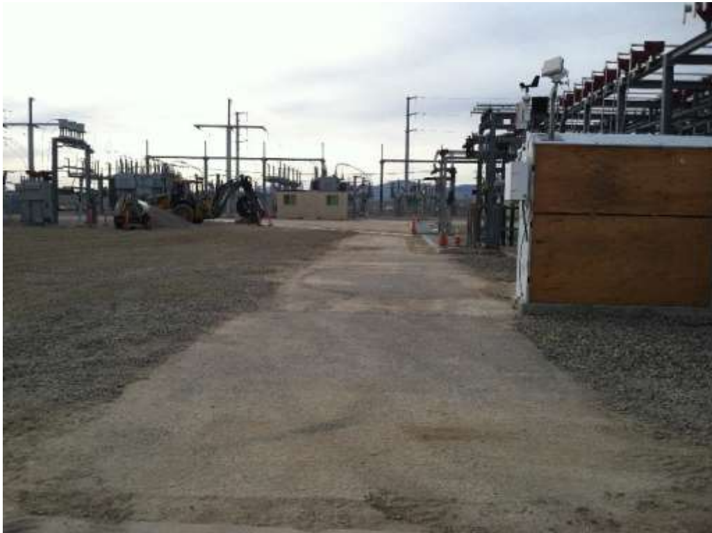
Figure 2 – Upcoming work will include resurfacing and extending asphalt driveways. View west, 02/22/16.
