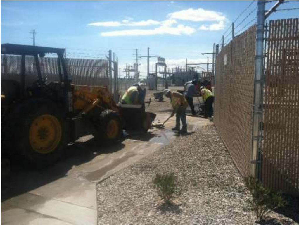
Figure 1 – Driveway paving activities occurred during the subject period. View southeast 4/12/16.
