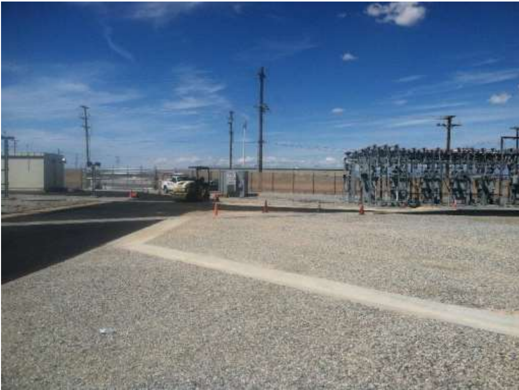
Figure 2 – Driveway paving activities were completed during the subject period. View north, 4/12/16.
