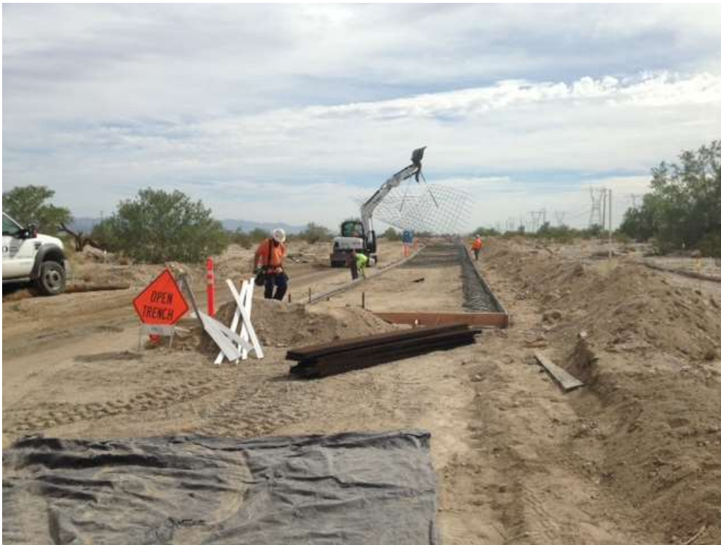
Figure 2. Construction personnel laying rebar forms for the Arizona crossings.
