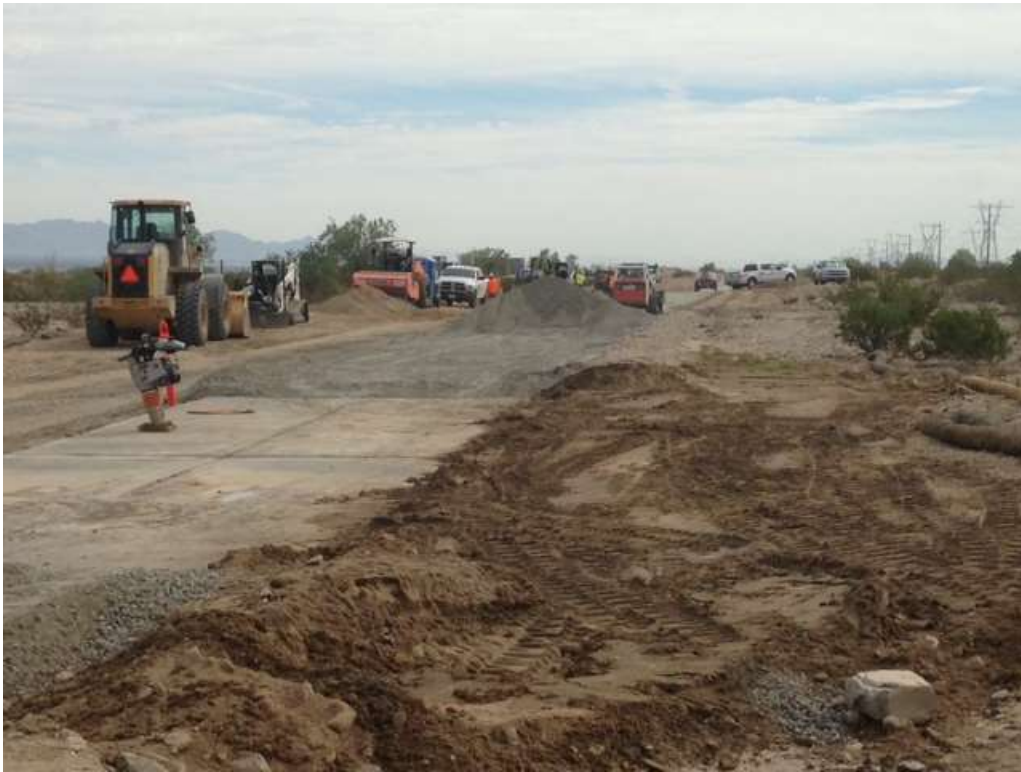
Figure 1. Construction personnel spreading rock along the Red Bluff access road.
