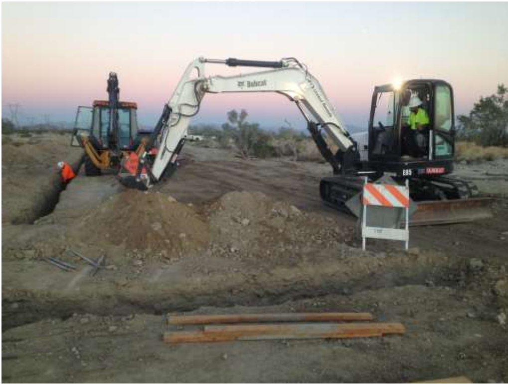
Figure 1. Construction personnel trenching Arizona crossings (photo courtesy of FRED).
