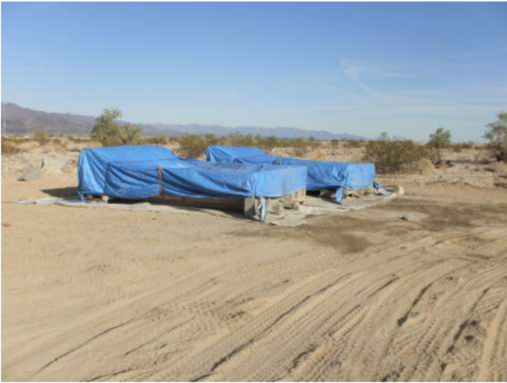
Figure 3. Properly contained concrete wash-out bins on the Red Bluff access road.
