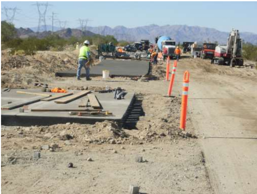
Figure 2. Concrete pouring for Arizona Crossings.
