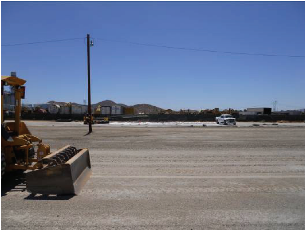
Figure 3: Construction activities occurring at the Menifee Construction Yard.
