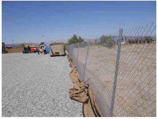
Figure 6: Fence damaged by wind along eastern boundary at DC2 Yard.
