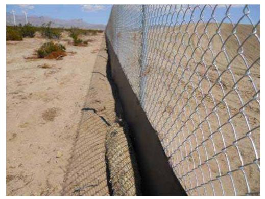
**Figure 6:** Existing silt fence along northern boundary of Devers Yard determined compliant with SWPPP conditions.
