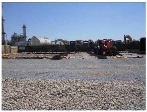
Figure 9: Secondary containment and protective netting being utilized at Menifee Construction Yard.
