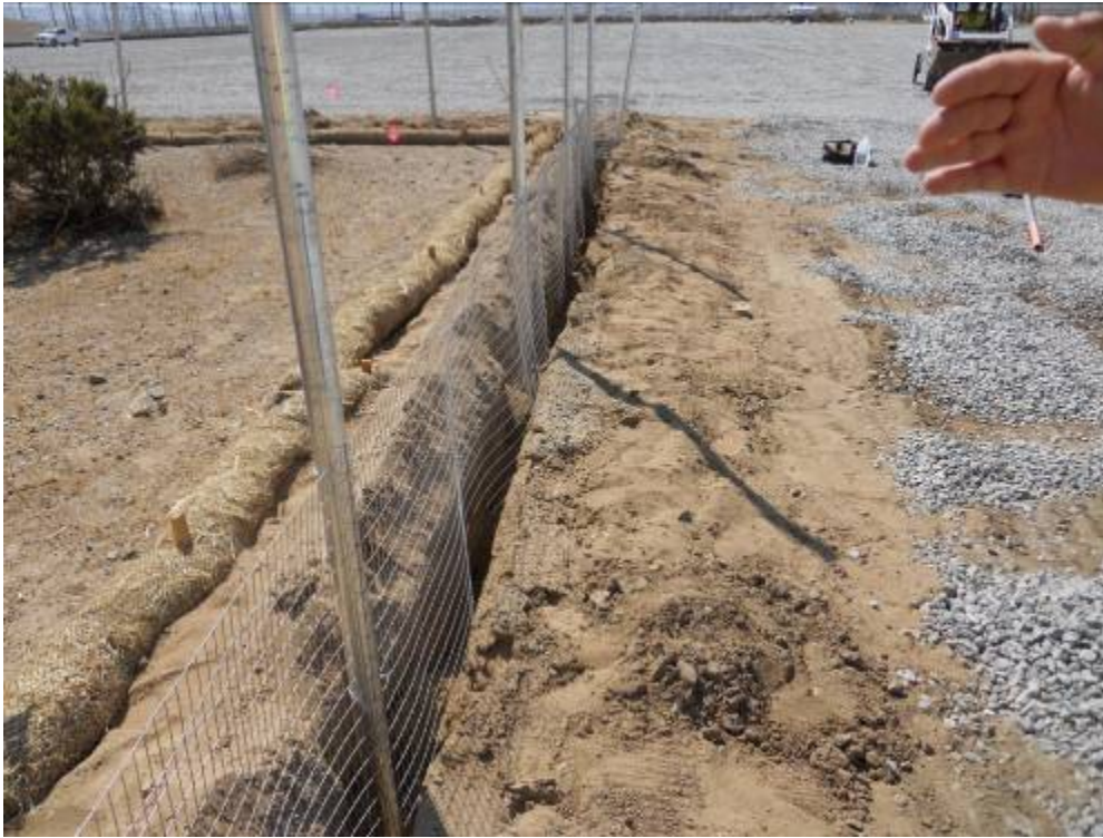
Figure 4: Trenching associated with desert tortoise fence installation at Devers Construction Yard.
