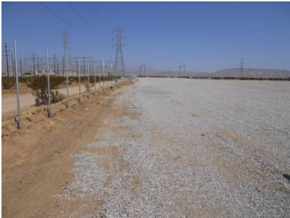
Figure 2: Fence installation activities at the Devers Construction Yard.
