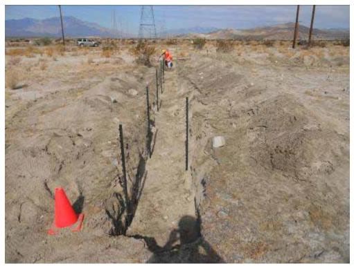
Figure 7: Trenching at exclusionary fencing locations.
