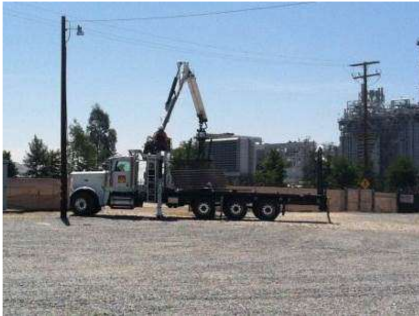
Figure 7. Shaker plate removal at the Meniffee Yard.
