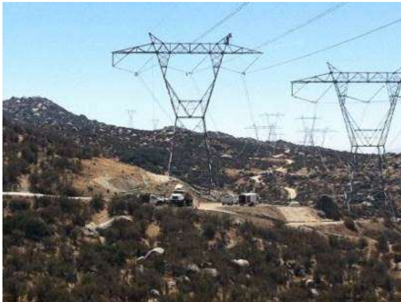
Figure 2. OPGW wire pull set-up at Tower 1137.
