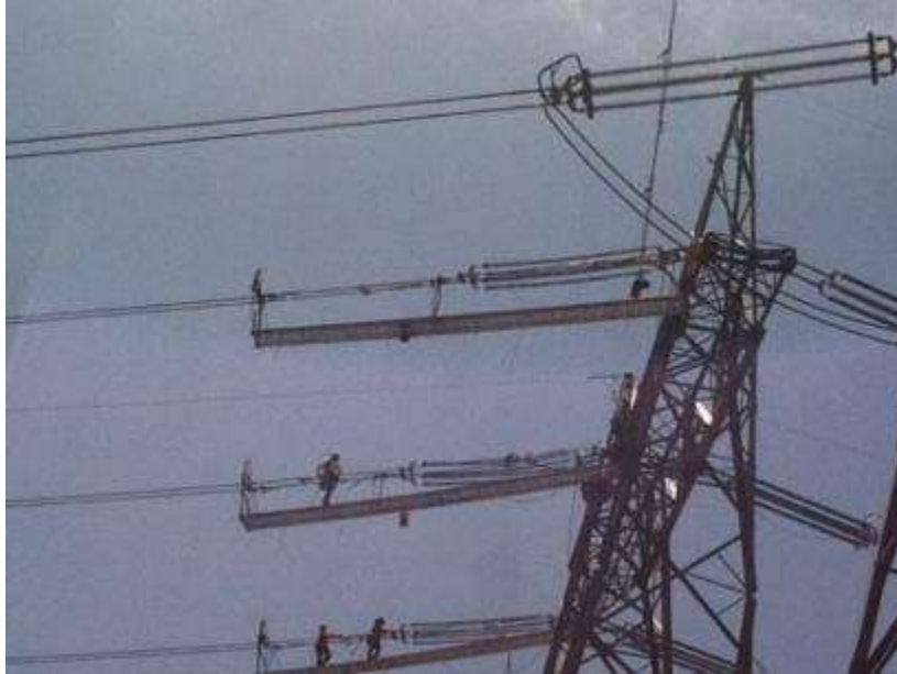
Figure 1. Dead-end conductor work at Tower 1141.
