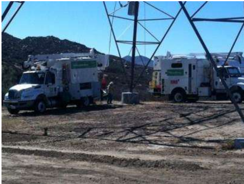
Figure 4. Telecomm splicing work at Tower 1094.
