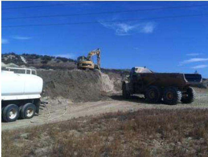
Figure 3. Site stabilization activities at Wire Site 36.
